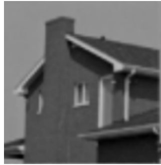
d. Original Building Image
