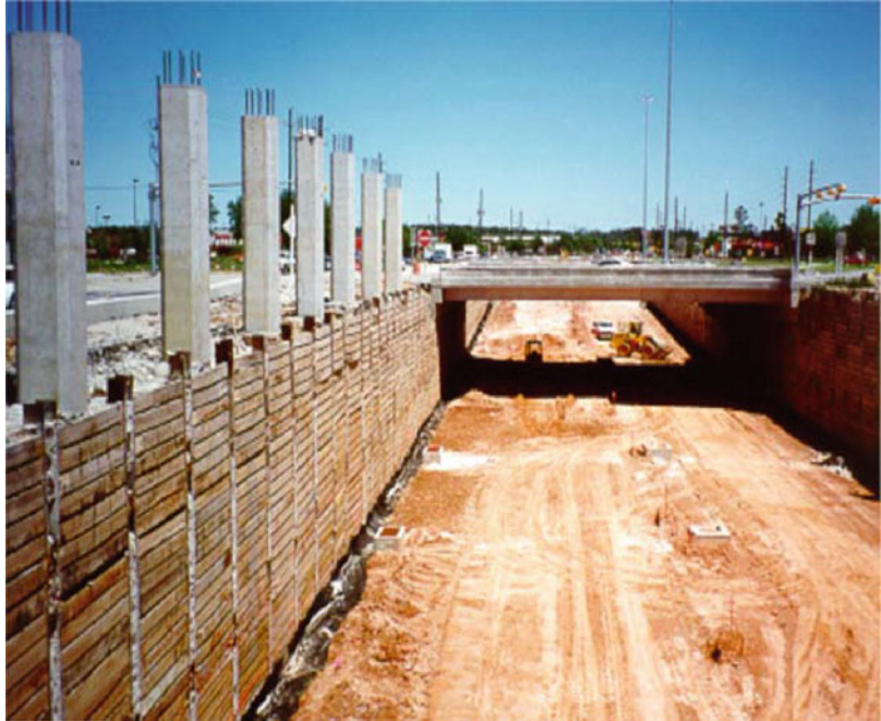
Analysis and Design Issues of Geotechnical Systems: Rigid Walls, Fig. 3 Braced excavation
