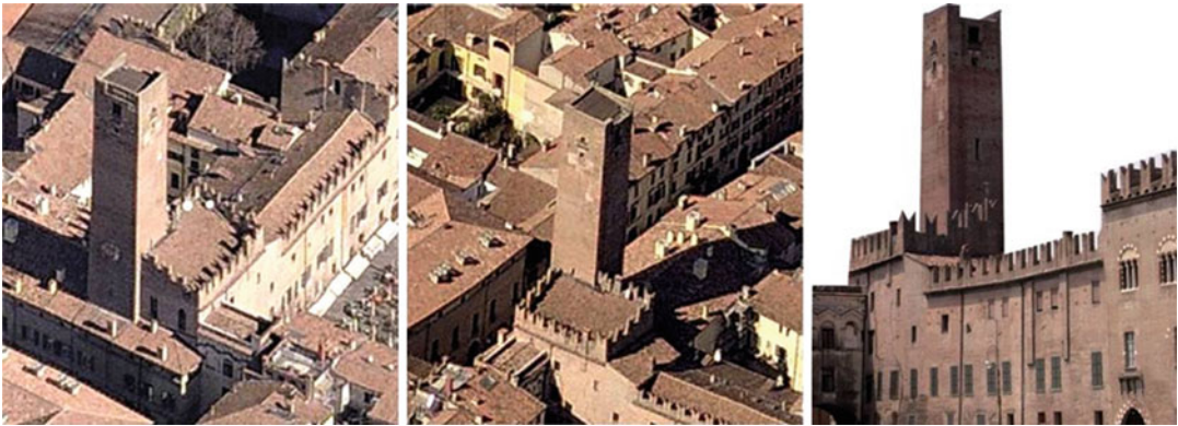
Ambient Vibration Testing of Cultural Heritage Structures, Fig. 9 Views of the Gabbia Tower (Mantua, Italy) from South and East
