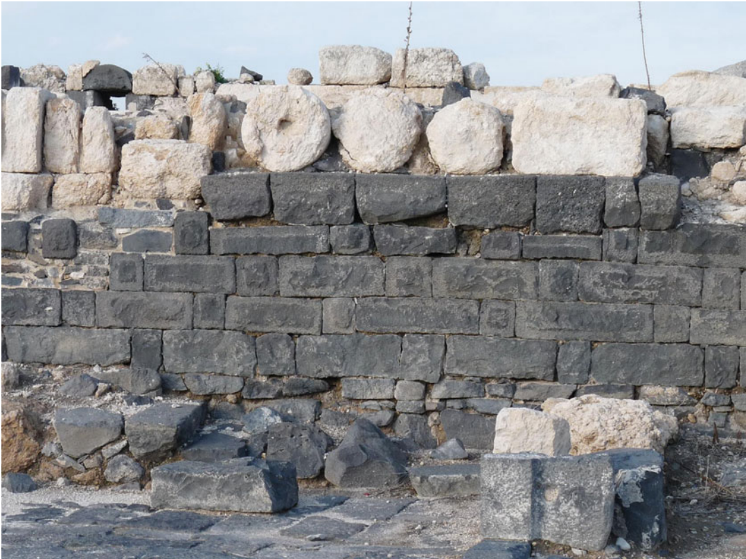
Archeoseismology, Fig. 5 Recycling of building material in repair works of a wall at Susita (Golan Heights) (cf. Sintubin 2011), possibly after a destructive earthquake © Sintubin
