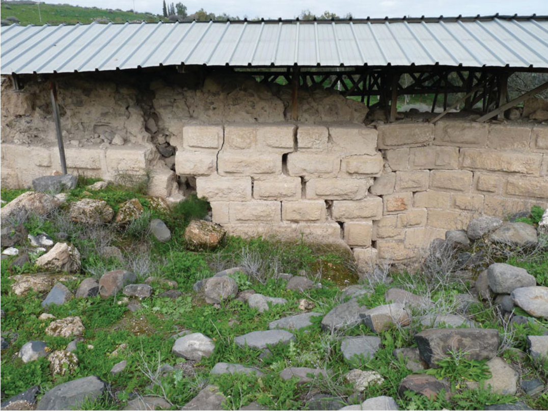
Archeoseismology, Fig. 2 The wall of the Crusader Fortress of Vadum Iacob (Ateret, Israel) (cf. Marco et al. 1997) is displaced left laterally over more than
