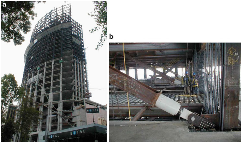
Buildings and Bridges Equipped with Passive Dampers Under Seismic Actions: Modeling and Analysis, Fig. 1 (a) Torre Mayor Tower under
