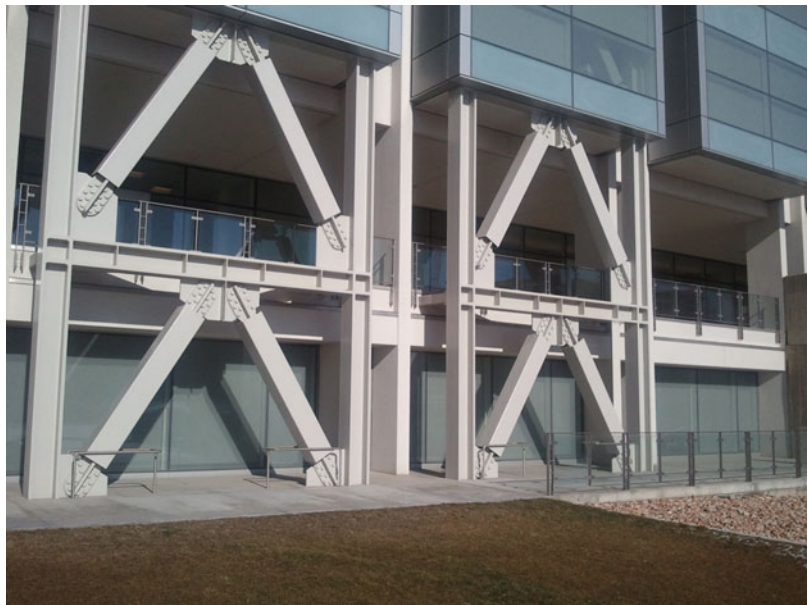
Fig. 4 Photograph of building retrofitted with BRBs (Courtesy of Core Brace, LLC)
