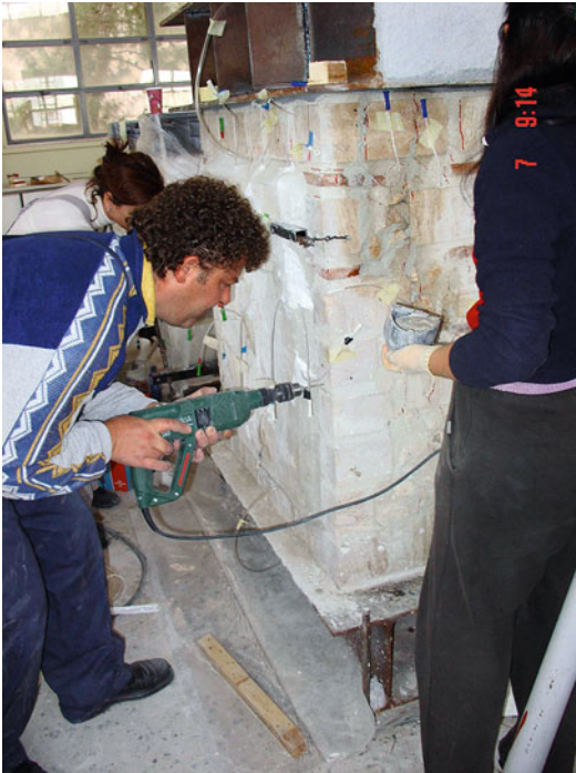
Strengthening Techniques: Masonry and Heritage Structures, Fig. 7 Drilling holes in masonry
