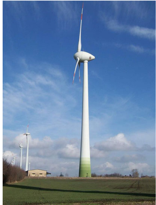
Seismic Analysis of Wind Energy Converters, Fig. 1 Horizontal axis wind turbine (HAWT) in Egel, Germany (photo by Hadhuey)
