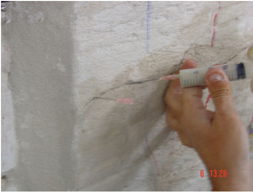
Strengthening Techniques: Masonry and Heritage Structures, Fig. 9 Sealing of cracks
