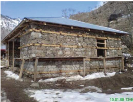
Seismic Analysis of Masonry Buildings: Numerical Modeling, Fig. 9 Bhatar construction: traditional unreinforced load-bearing timber-laced masonry structure in Pakistan in modern construction (Source: http://www.holcimfoundation.org/Projects/advocacy-of-traditional-earthquake-resistant-construction-north )
