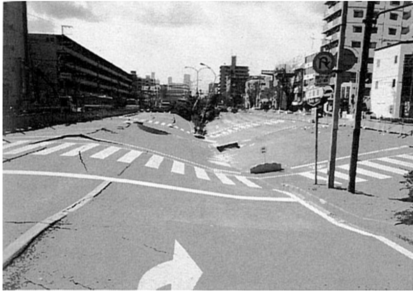
Seismic Design of Tunnels, Fig. 2 Street view of Dakai subway station collapse (Iida et al. 1996)
