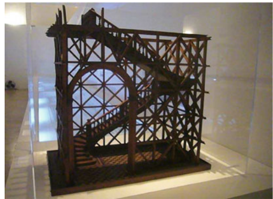
Seismic Analysis of Masonry Buildings: Numerical Modeling, Fig. 10 Model of the Gaiola pombalina masonry confinement with timber, developed in Lisbon after the 1755 earthquake ( http://en.wikipedia.org/wiki/Gaiola_(construction) )
