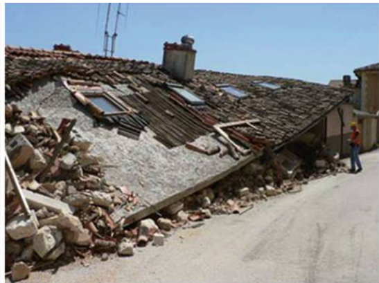
Strengthening Techniques: Masonry and Heritage Structures, Fig. 21 Catastrophic effects of RC slabs supported by poor-quality masonry (Courtesy of Prof. C. Modena)
