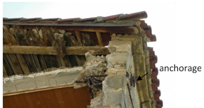
Strengthening Techniques: Masonry and Heritage Structures, Fig. 25 Elaborate connection between walls at the corners of masonry buildings
