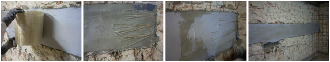
Seismic Strengthening Strategies for Heritage Structures, Fig. 4 Corner confinement of masonry walls by use of SRP strips anchored with SRP connectors (Photo Paolo Casadei 2008, product FIDSTEEL)
