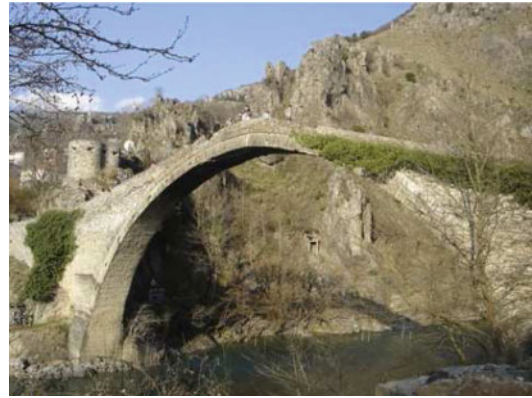
Seismic Analysis of Masonry Buildings: Numerical Modeling, Fig. 4 The Aaos river bridge (eighteenth century), Hepirus, Greece
