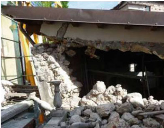
Strengthening Techniques: Masonry and Heritage Structures, Fig. 21 Catastrophic effects of RC slabs supported by poor-quality masonry (Courtesy of Prof. C. Modena)
