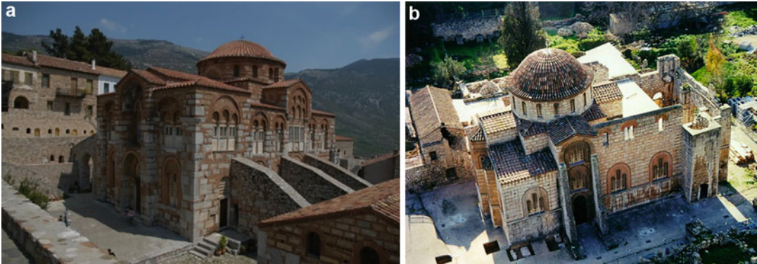
Strengthening Techniques: Masonry and Heritage Structures, Fig. 34 (a) Ossios Lucas Monastery: external stone masonry buttresses were added against the southern facade. Due to architectural constraints, the buttresses do not reach the critical region of the system of arches that support the cupola. (b) Dafni Monastery:
