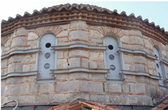
Strengthening Techniques: Masonry and Heritage Structures, Fig. 33 Dafni Monastery: existing steel tie at the base of the cupola, to be replaced by a stainless steel tie
