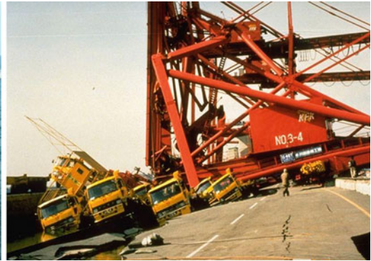
Seismic Vulnerability Assessment: Lifelines, Fig. 8 Failure of port infrastructures in 1995 ( M_w 6.8) Hyogoken–Nanbu earthquake (Photo by K. Pitilakis)
