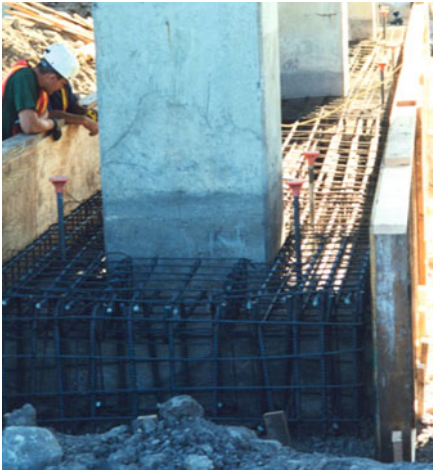
Strengthening Techniques: Bridges, Fig. 11 Footing strengthening using grade beam and pile cap to pile steel bars
