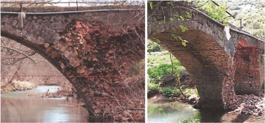
Strengthening Techniques: Masonry and Heritage Structures, Fig. 29 Partial collapse of the bridge after the passage of a heavy track
