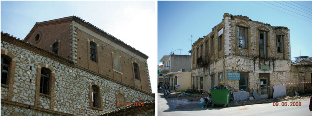
Strengthening Techniques: Masonry and Heritage Structures, Fig. 25 Elaborate connection between walls at the corners of masonry buildings
