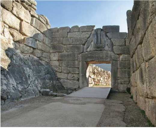
Seismic Analysis of Masonry Buildings: Numerical Modeling, Fig. 1 The stone masonry castle of Mycenae, Peloponnese, Greece, 2nd millennium BC (Source http://en.wikipedia.org/wiki/Mycenae )
