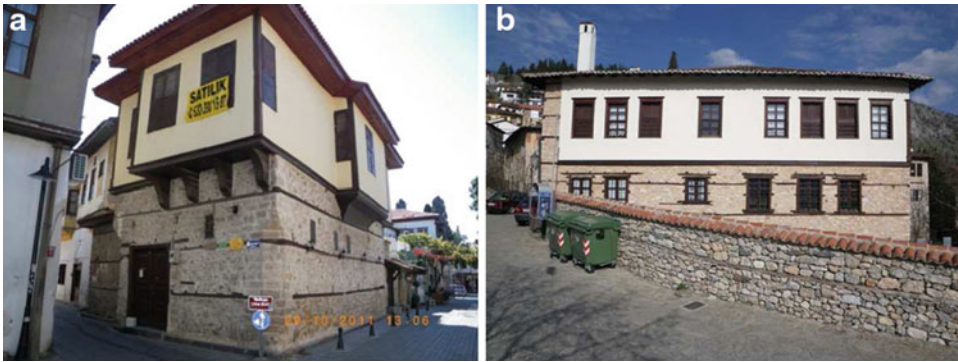
Seismic Analysis of Masonry Buildings: Numerical Modeling, Fig. 8 Traditional timber-laced stone masonry buildings in earthquake-prone areas. (a) Antalya, Turkey. (b) Kastoria, Greece
