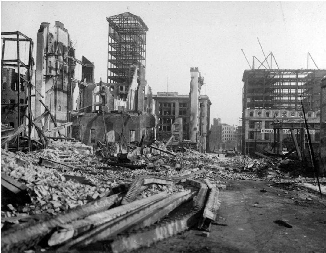
Steel Structures, Fig. 5 Damaged buildings from the 1906 San Francisco earthquake and fire. The two tall steel frames were under construction and were not damaged.
