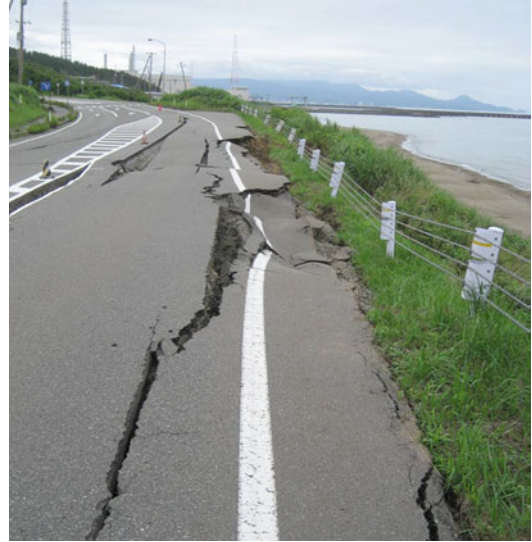
Seismic Vulnerability Assessment: Lifelines, Fig. 4 Damages to road embankments in 2007 Niigata-Chuetsu Oki ( M_w 6.6) earthquake (Photo Credit: US Geological Survey)
