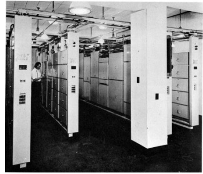
Fig. 5.4. BELL Relay Calculator, designed by Stibitz
