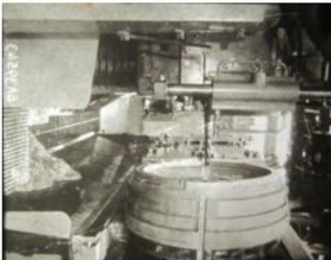
2: Cutting starts on the rough cuts
