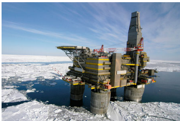
Fig. 2 Oil and gas platform in the ice cover
