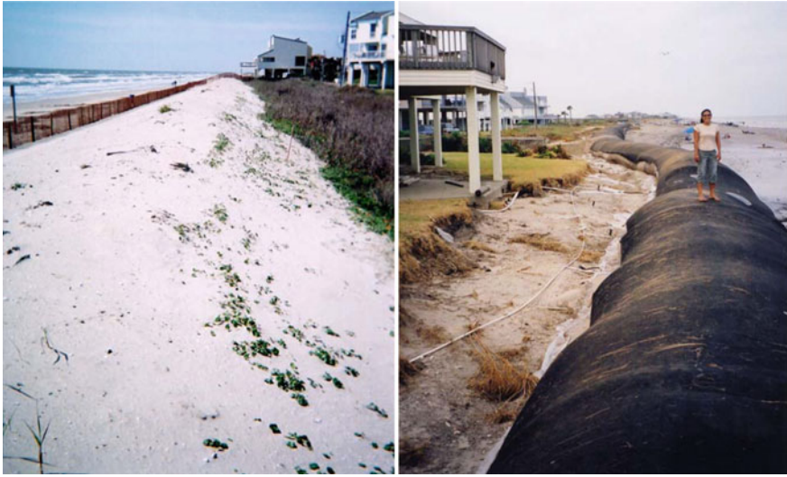
Fig. 6.1 Foredune restoration project at the Pirates' Beach. Left image shows the geotube covered with sand, prior to planting vegetation. Right image shows the geotube after Hurricane Lilly removed the sand and vegetation in 2002. By 2003, the geotube was partially torn apart by Hurricane Claudette. Photos by Rusty Feagin
