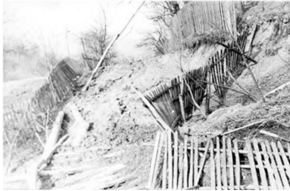
Fig. 4 Fans damaged by toe of landslide, in Slon, Prahova County, after the 1977 earthquake [4]
