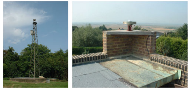
Fig. 16.1 HERS (top of tower) and HERT GNSS sites
