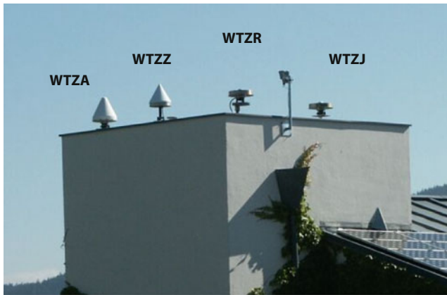
Fig. 20.1 GNSS permanent sites on top of the tower of the main building of the Geodetic Observatory Wettzell. A webcam to monitor snow coverage of the antennas is mounted between WTZR and WTZJ
