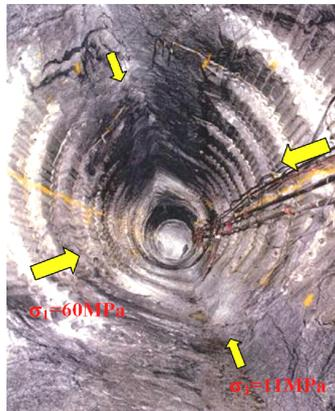
Fig. 2. Notch breakouts occurred at the Mine-by tunnel [15]
