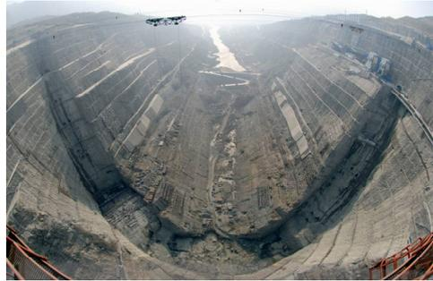
**Fig. 13.** Unbalance force summation at dam toe for anchorage design **Fig. 14.** An overall view of the foundation excavation of Xiluodu arch dam
