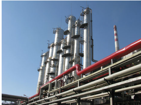
Fig. 4.5 Butanol acetone distillation tower [39]
