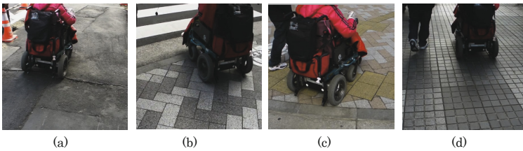
Fig. 7. Examples of ground surface with mobility barriers (a) rough road surface, (b) sidewalk curbs, (c) tactile surface indicator, (d) tile paving with rough joint
