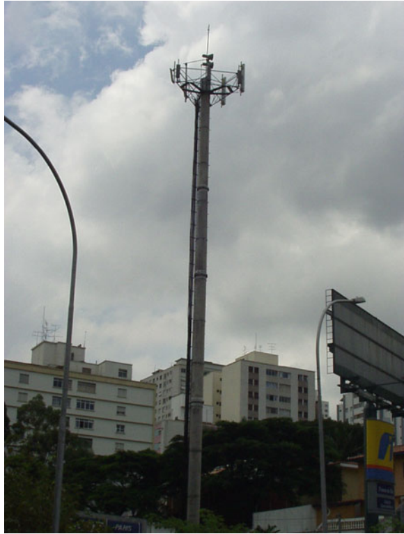
Fig. 1 Typical pre-cast RC telecommunication tower
