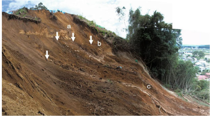
Photo 33.3 Displaced slope (AA' cross section) a Volcanic ash deposits, b Pyroclastic debris deposits, c unconsolidated gravels arrows: outlets of groundwater discharge (springs)
