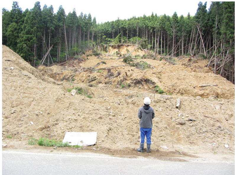
Fig. 73.2 Whole view of the landslide
