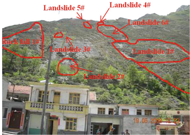
Fig. 37.1 General view of the FaTing mountain landslide
