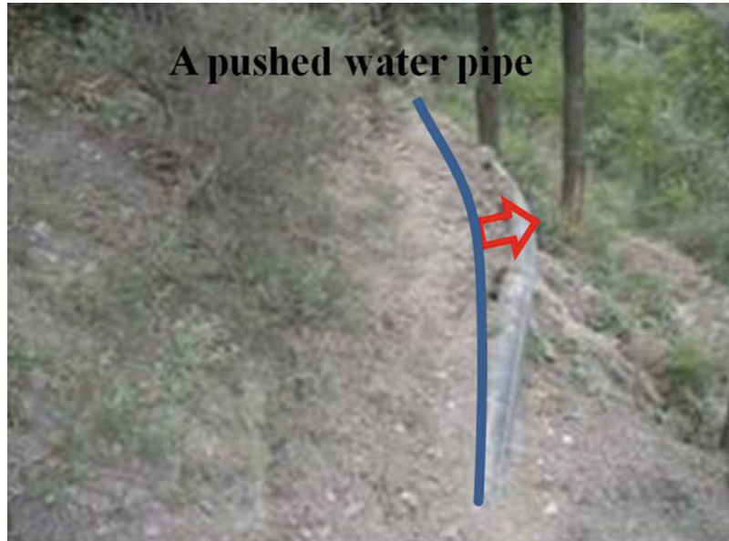
Fig. 37.5 Pushing trace of the water pipe
