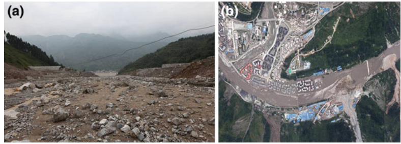
Fig. 103.4 a The destroyed check dam in Qingping debris flow; b Ming river blocked at Yingxiu town by Hongchungou debris flow (photographs from Tang chuan)
