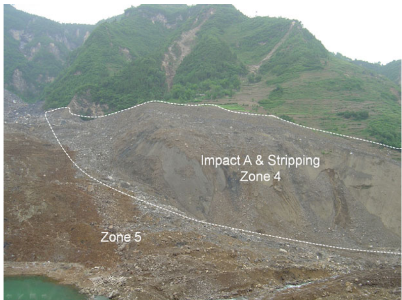
Fig. 51.4 Impact A and stripped surface of second slope opposite first slope over a V-shaped stream course of Donghekou rockslide-debris flow
