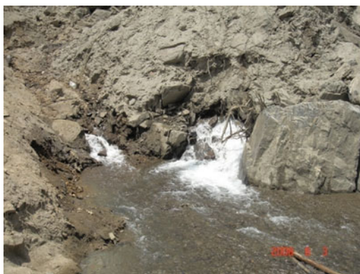
Fig. 105.5 An overflow points at 669 m elevation of Tangjiashan barrier dam's downstream slope toe
