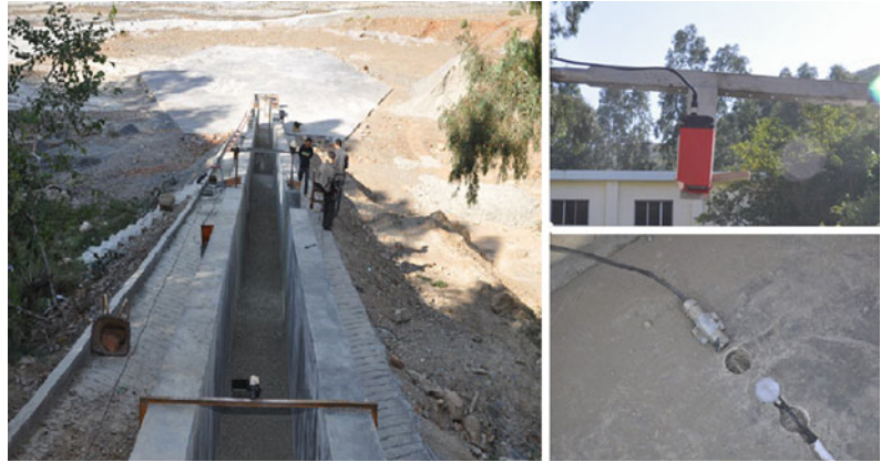
Fig. 99.2 Experimental installation: a the distribution of landslide dams in the experimental flume; b an instrument for measuring the depth of debris flow; c pore water pressure sensors and total stress sensors
