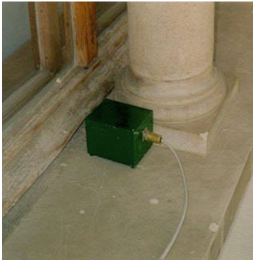
Fig. 96.7 Place of installation of BKPI-2 M sensor of inclination angles and vibrations on the south-eastern part of the Livadia Palace
