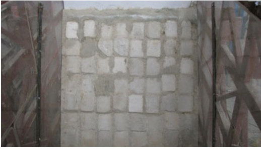
Fig. 7.9 Building with solid blocks
