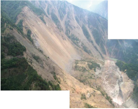
Fig. 54.7 Overview of the Tangjiashan landslide, Beichuan
