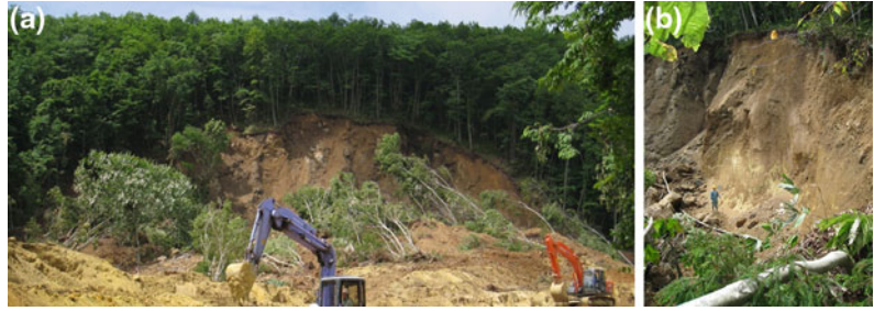
Photo 45.2 Views of the Hikagemori landslide. a debris slide, b head-scarp
