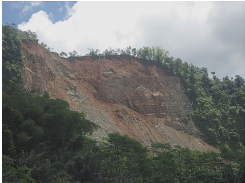
Fig. 26.3 Overview for the induced landslide (major affected parts)
