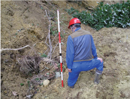
Photo 45.5 Easily-liquefied soils exposed at the run-out area of the Hikagemori landslide
