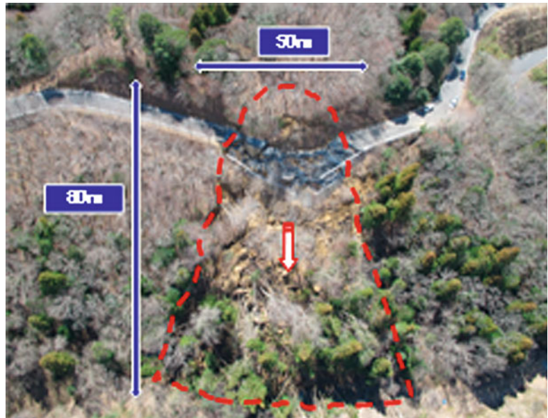
Fig. 28.6 Bird's eye view of the Morosawa landslide
