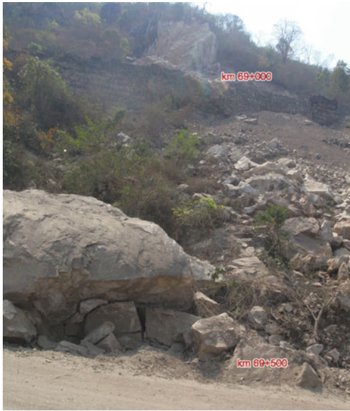
Fig. 4.2 An overview of Bhedetar landslide
