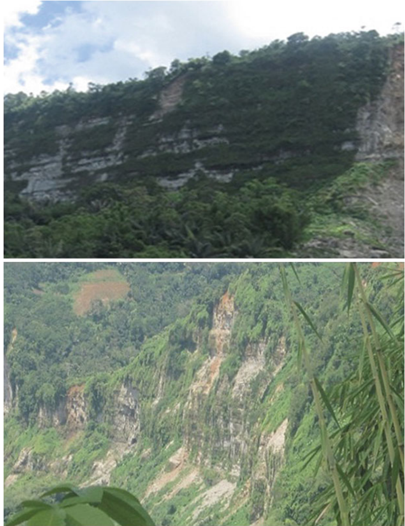
Fig. 26.4 Examples for the shapes of natural slopes in the Clicangkareng landslide area
