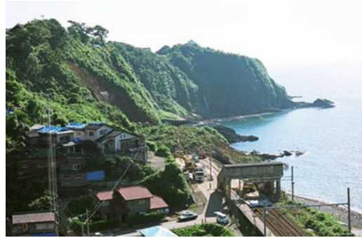
Photo 8.5 Landslide close to the Omigawa railway Station caused by the Niigata-ken Chuetsu-oki Earthquake (2007) (Niigata Pref., Japan) (taken by Sakurai M.)
