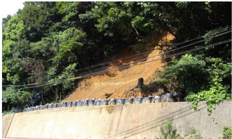
Fig. 93.12 Occurrence of larger size of slope failure next to former small failure
