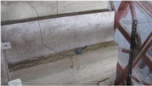
Fig. 7.10 Building layer by layer
