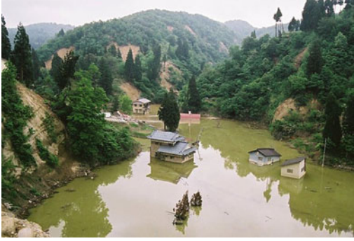
Photo 8.1 Submerged village and road by landslide dam caused by the Mid Niigata Prefecture Earthquake in 2004 (Higashi-Takezawa village, Niigata Pref., Japan) (Sakurai and Goto 2005)
