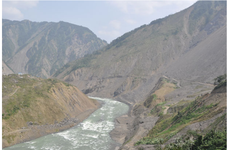
Fig. 98.2 An armoring layer rough layer with coarse material in the surface of spillway in the Tangjiashan dam after breaching
