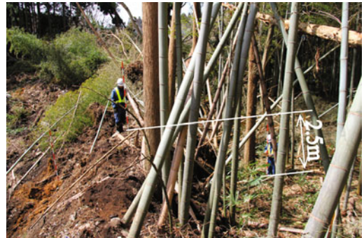
Photo 30.3 Colluvial soil deposited on one side cliff of the depression
