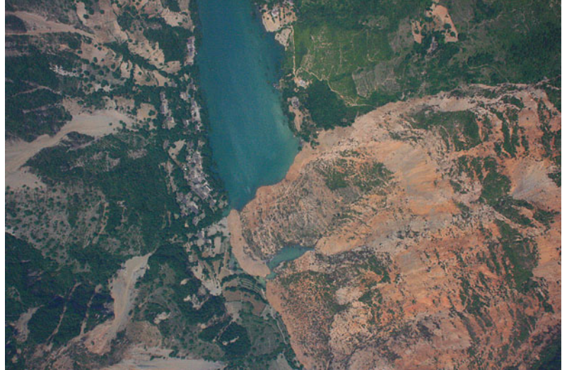
Fig. 18.2 Aerial photograph of Wenjiaba landslide
