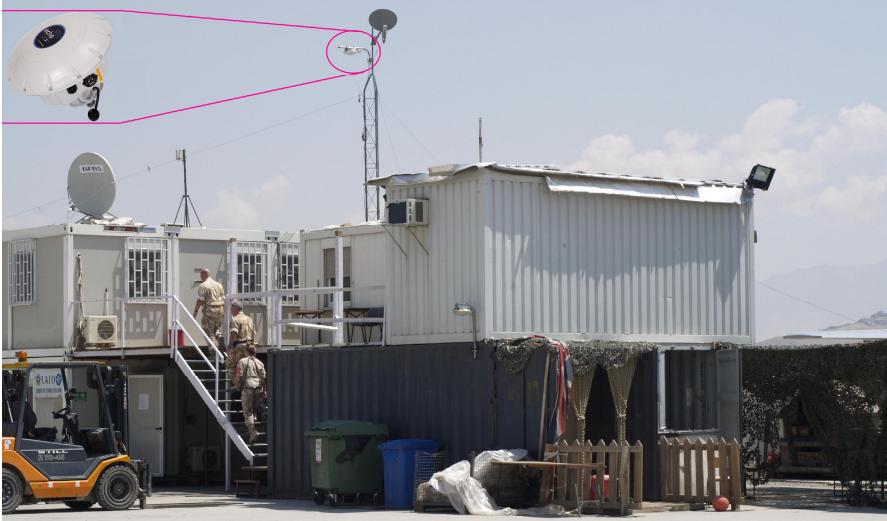
Photo 2.1 NATO Consignment Tracking by LOG– the antenna on the building collects RFID-data (Picture: LOG)
