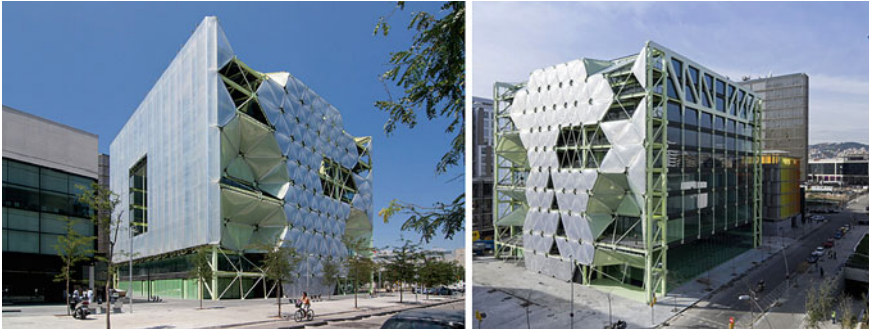
Fig. 1 Views of the Media-TIC building. Left: SE and SW façades; Right: SE and NE façades. Credits: José Miguel Hernandez, Iwan Baan
