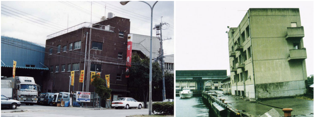
Fig. 7 Building failures after the 1995 Kobe earthquake
