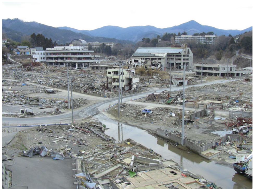
Fig. 1 Devastation of a Coastal City during Japan Earthquake 2011 [Photo courtesy Dr K.Goda]
