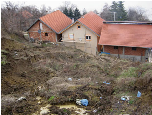
Fig. 2 Landslide Vinča (Photo December 2009)
