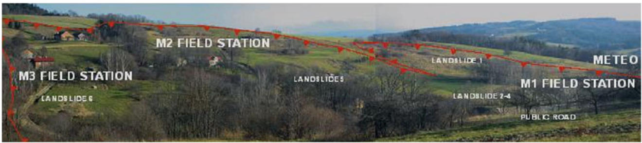
Fig. 2 Place of real-time monitoring system installation
