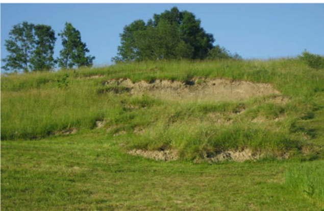
Fig. 7 New cracks (May 2010) – central part of landslide no 5
