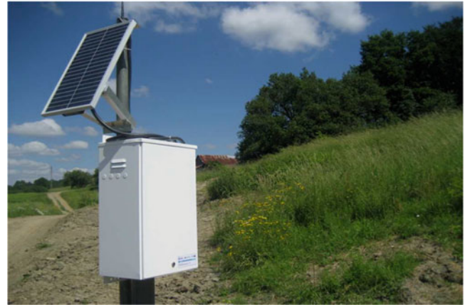
Fig. 13 M2 Field Station on landslide no 5
