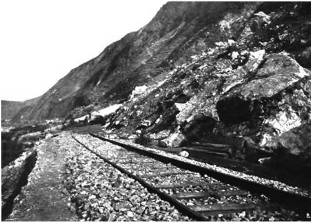
Fig. 5 Rockslides and rockfalls occurred along the railway line in Favazzina (Società Fotografica Italiana 1909)
