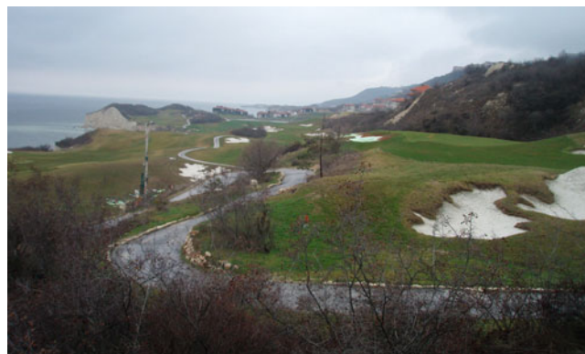
Fig. 3 Kalkantepe landslide, between Balchik town and Kavarna town
