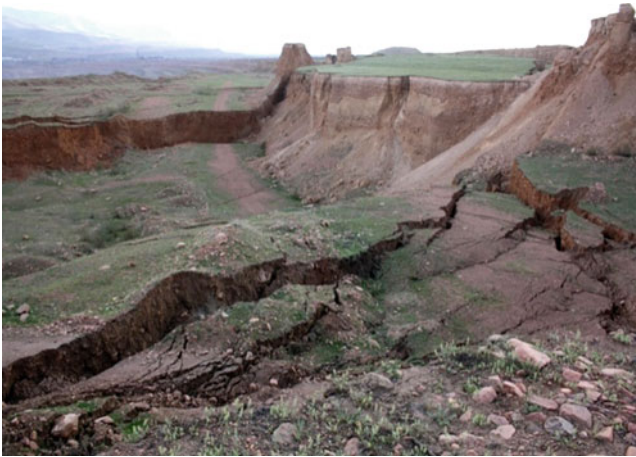
Fig. 5 Down warping of upper part of landslide Old substation
