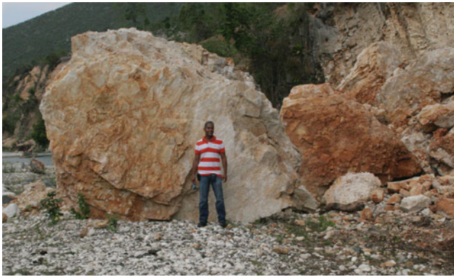
Fig. 2 Rock fall comprised of limestone boulders that have failed along preexisting fractures
