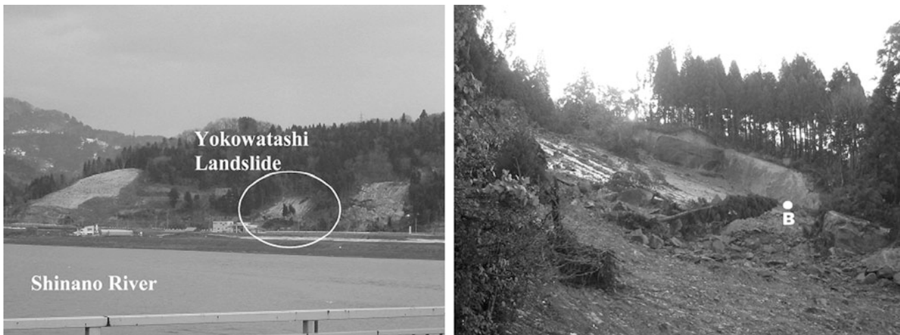
Fig. 3 Photos for the Yokowatashi landslide occurred at the time of The 2004 Mid Niigata Prefecture Earthquake in Japan (Point B in the right photo indicates the soil sampling point)
