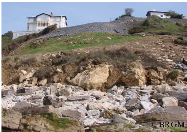
Fig. 8 Construction of a draining blanket over slid materials
