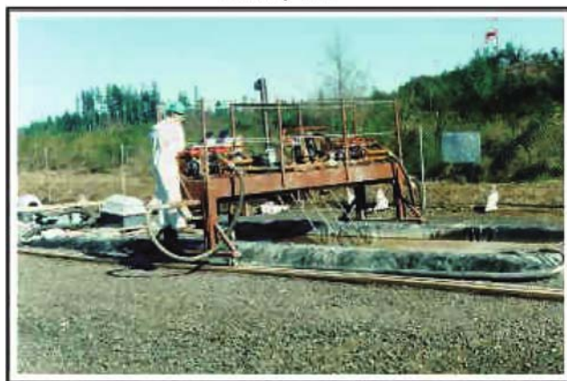
40 Cubic Yard Demonstration
