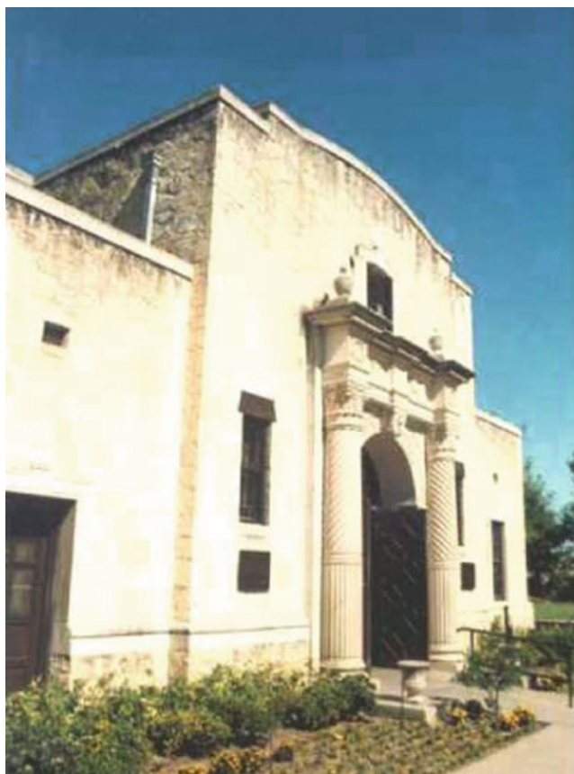
■ Fig. 12.22 Microbial adhesion and consequent deterioration only occurred at the top (dark) part of the building. The lower protected portion was free of bacteria and deterioration
