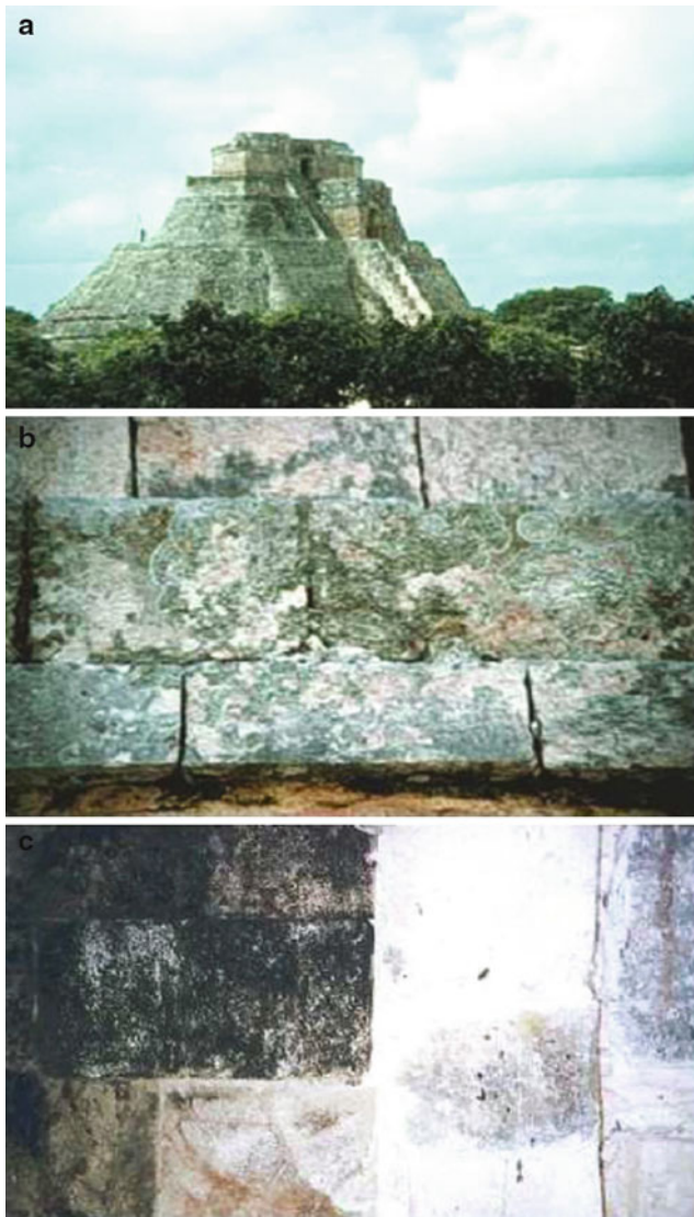
■ Fig. 12.2 Photographs showing (a) an ancient Mayan temple made of limestone covered by microbial biofilms, (b) a close-up view near the base, and (c) the contrast between newly replaced and original stone
