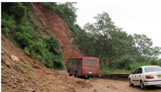
Fig. 4 A roadside landslide that occurred in the beginning of 2011
