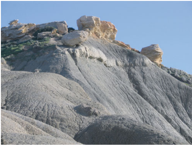
Fig. 7 Hazardous situation south of Il-Qarraba promontory due to the presence of limestone blocks in critical stability conditions. It should be noted that the blocks are overhanging footpaths and beach areas
