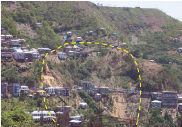
Fig. 5 Settlements in an old landslide area
