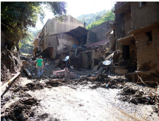
Fig. 2 Damages after the October 1, 2009 event in Briga village
