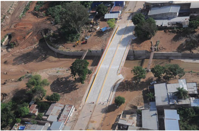
Fig. 15 New Packham Avenue bridge
