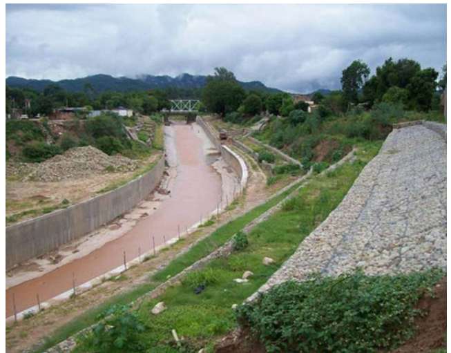
Fig. 8 Upstream view of Tartagal River channel in 2007. In the background the Packham Avenue bridge and the railway bridge can be seen
