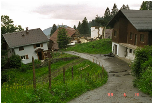
Fig. 3 Damaged houses in the village Rindberg (WLV GBL Bregenz)
