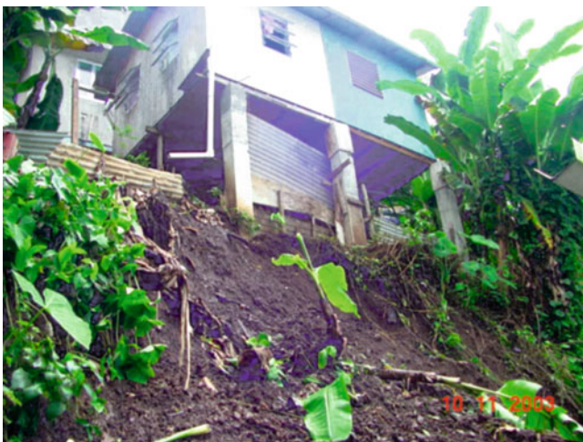
Fig. 4 Houses built on deep residual soils on steep slopes are vulnerable to landslides triggered by major rainfall events
