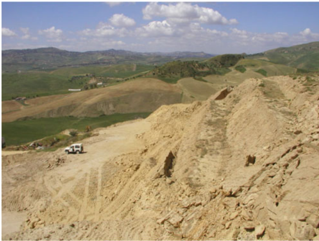
Fig. 8 The entire quarry face has collapsed with a shift of about 20 m (Photo M. Collalti Department of Energy – Geological and Geophysical Service IX Sicilian Region)
