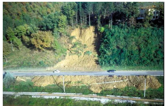
Fig. 3 Landslide near Loro Ciuffenna (AR), in the eastern side of Arno river basin
