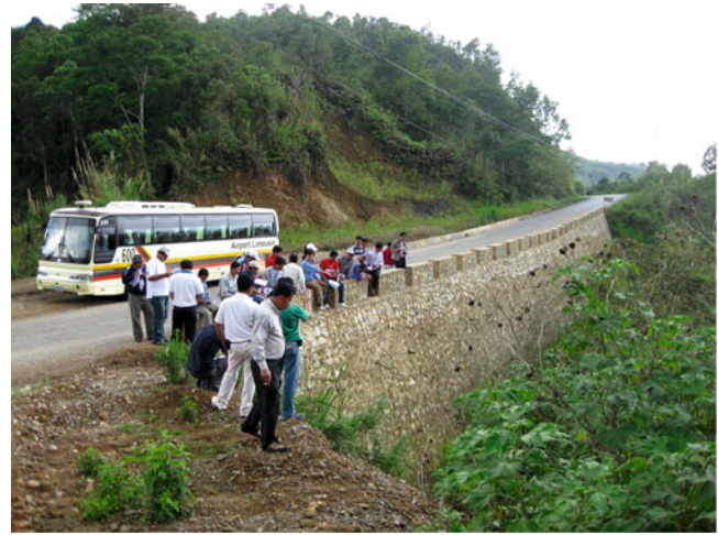
Fig. 5 Inspection of cemented masonry retaining wall
