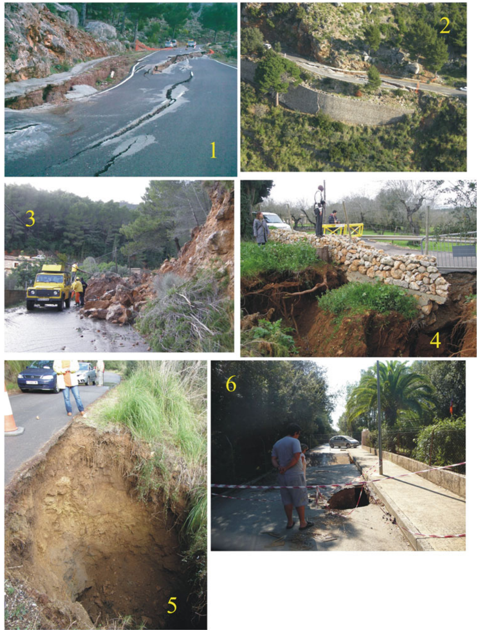
Fig. 3 Photographs of secondary roads on the range affected by landslides and karstic collapses (sinkholes). 1 and 2 Cala Tuent landslide (15/12/2008), 3 Es Verger landslide (15/12/2008), 4 Búger sinkhole (Jan 2010), 5 Es Verger sinkhole (15/12/2008) and 6 Crestatx sinkhole (3/5/2010)
