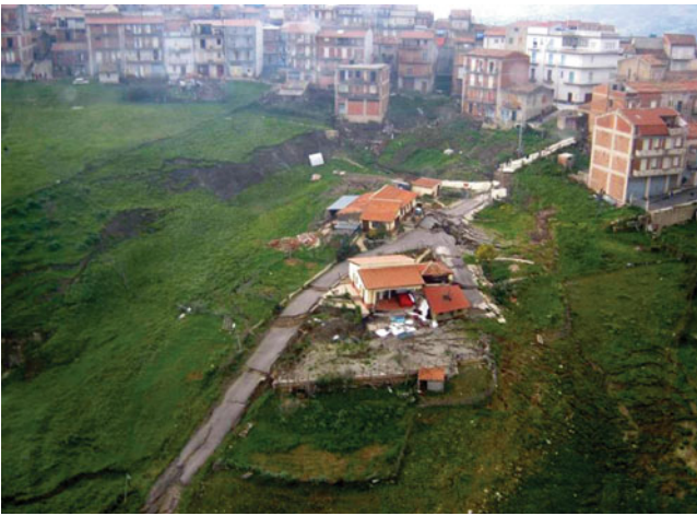
Fig. 8 The village of San Fratello (ME, Sicily) damaged by a landslide, February 14, 2010
