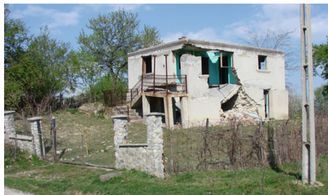
Fig. 3 Photograph of a household (2006), located on a stairstep, which was moved 8 m towards east (see Fig. 1)
