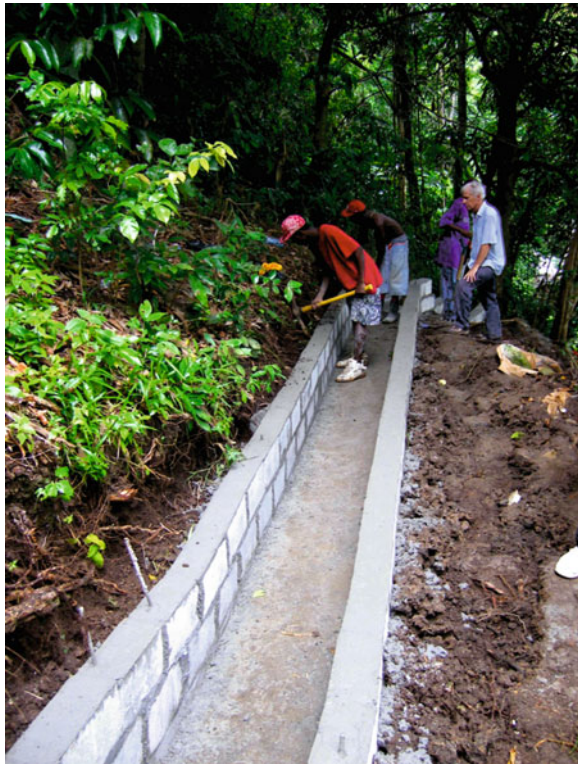
Fig. 5 Providing effective surface water management on slopes, rather than retaining structures (Fig. 2), can be an effective way of reducing landslide risk
