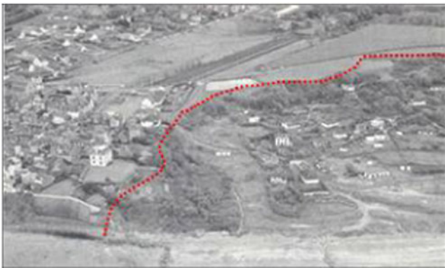
Fig. 4 East part of the main scarp of the Cirque des Graves landslide in 1982. On the toe of the landslide, several houses and tourist accommodation, now completely destroyed
