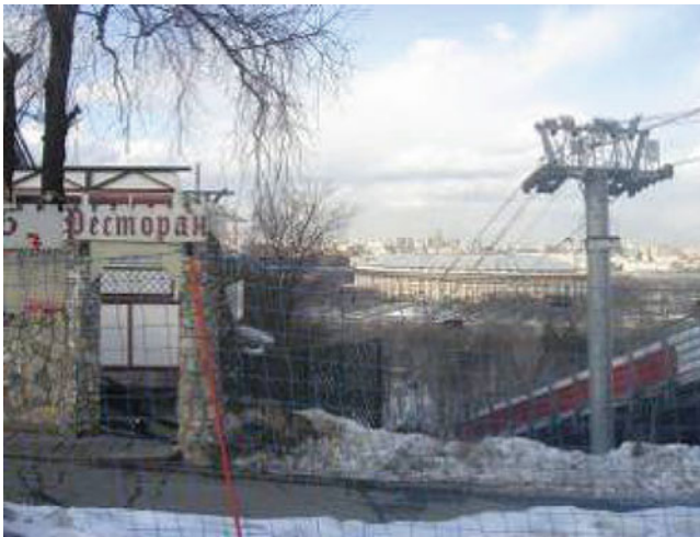
Fig. 6 Place of landslide activation near ski jump
