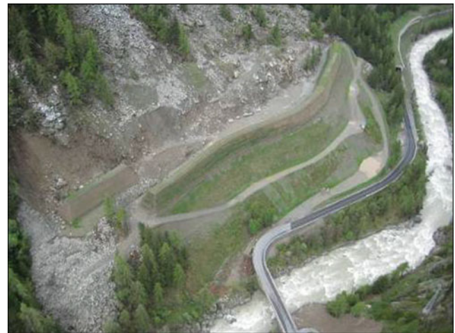
Fig. 14 Embankments built along the SR 47 (291 m and 50 m long)
