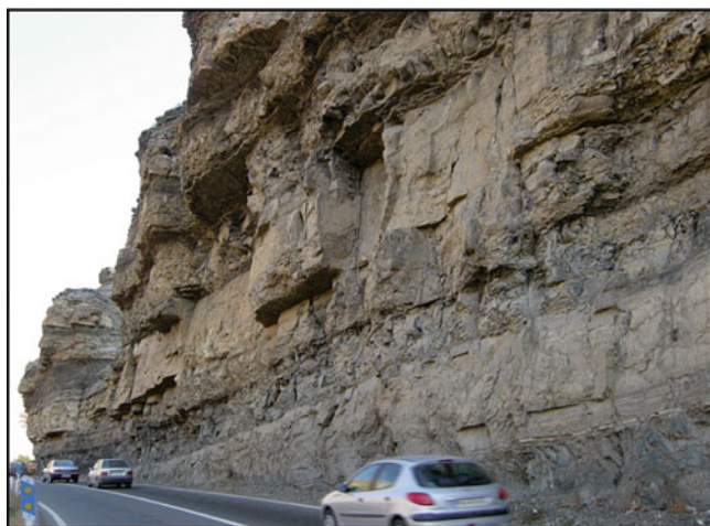
Fig. 3 Road-cut through Tuffaceous rocks of Karaj formation and development of rock falls
