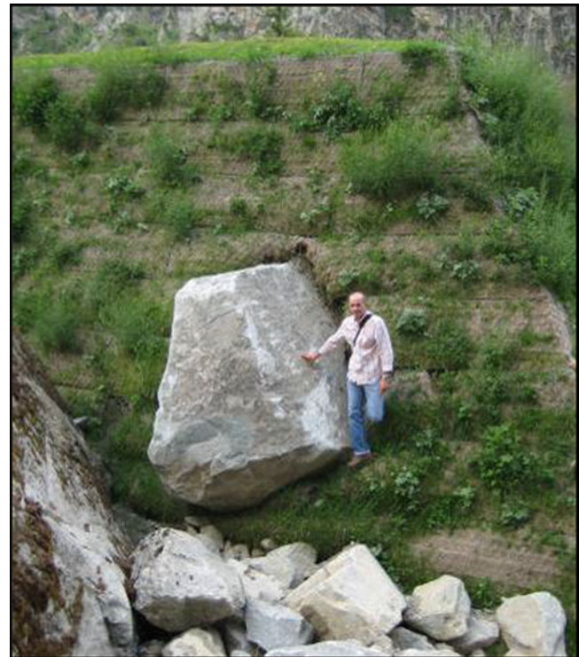
Fig. 10 Block impacted against the GTM embankment and used on the back analysis
