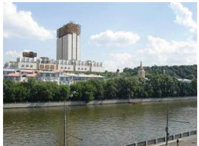
Fig. 4 Presidium of RAS, Andreevsky monastery and new buildings on landslide slope
