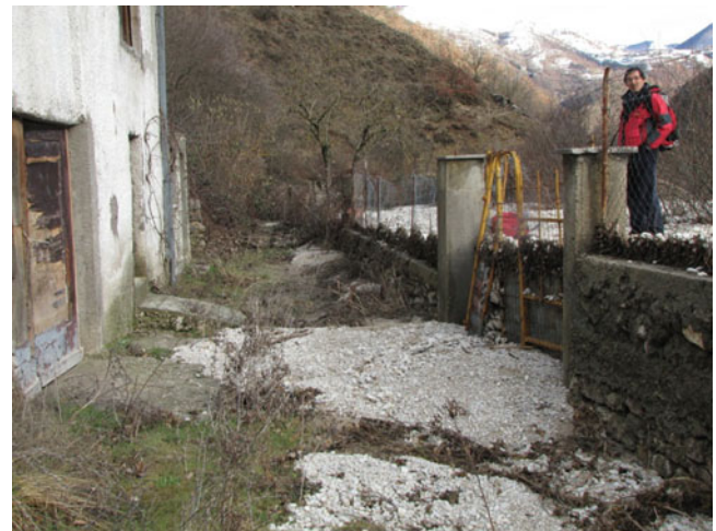
Fig. 4 Overflowing of the external areas of the riverbed of the Scura Valley, alluvial event of the last 1st and the 2nd of December (2010)
