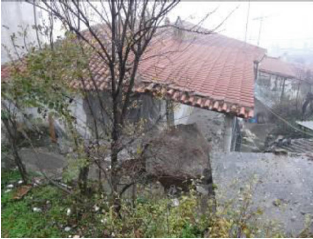
Fig. 4 Damaged house and the boulder of the 19 December 2010
