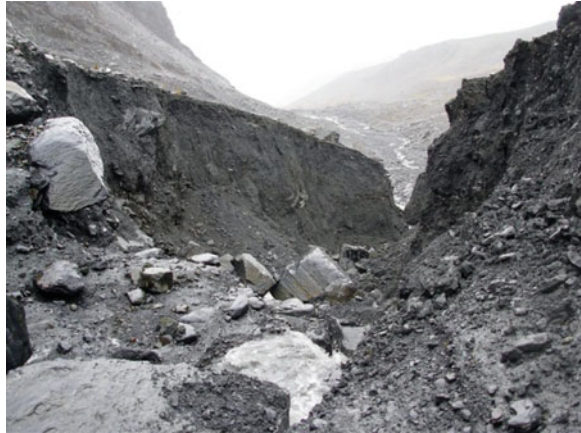
Fig. 5.5 Breach in the moraine dam below the glacial lake ( Source Martín Apaza Ticona, 4 November 2009)
