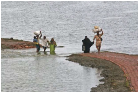
Fig. 15.7 Damaged road ( Source The Daily Star Newspaper, Monday, 1 June 2009)
