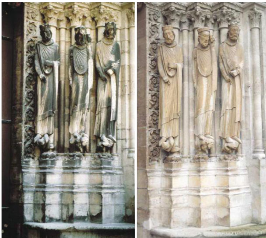
Fig. 6.71 Laser cleaning of a portal at Sant Denis Cathedral in Paris [83]
