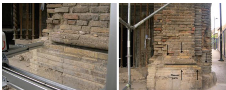
Fig. 6.72 Automated 1064 nm, 5 ns pulse width Laser cleaning of a brick pillar on the façade of the Cathedral in Tarazona (Spain) [84]
