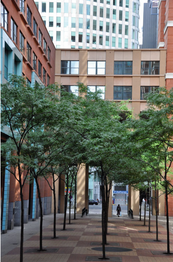
Fig. 6.7 These trees can only grow between high-rise buildings and on top of a car park because of an underground structure
