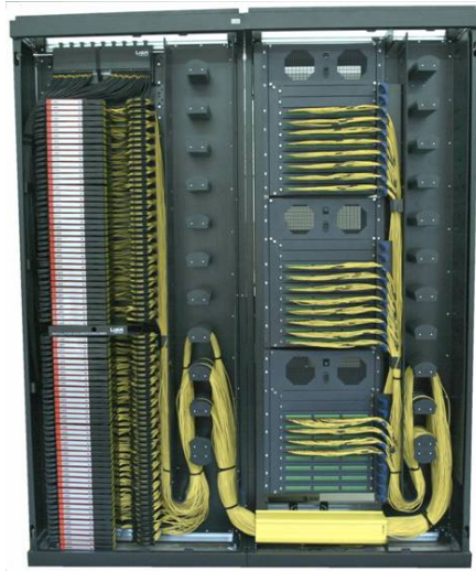
Fig. 3. High-density fiber management solution (source: Huber&Suhner)
