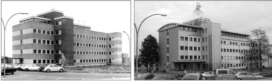
Fig. 51.5 IPA building at DVL/DLR research center in Oberpfaffenhofen. Left: spring 1968 shortly after completion with 1.4-m dish of a precipitation radar on the roof, also containing offices of other DVL branches. Right: January 2012, renovated with new entry pavilion, extended 5th floor and 5.5-m dish of POLDIRAD on the roof, occupied solely by IPA staff
