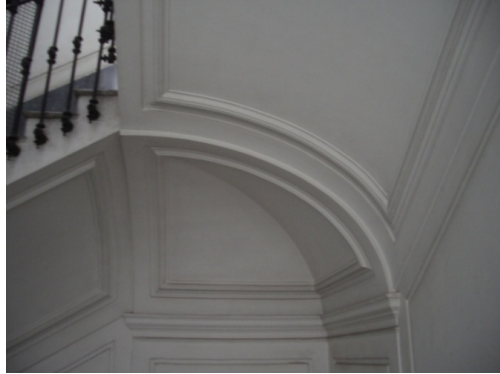
Fig. 6.2. Stair corner at the flight-to-landing intersection
