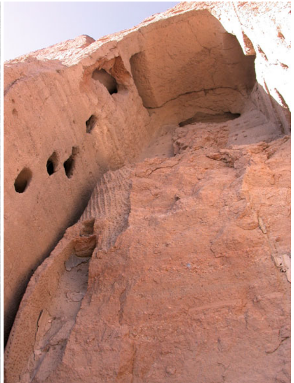
Fig. 9.5 Pattern of discontinuities in the Eastern Giant Buddha niche both before intervention of the Indian Archaeological Survey and currently (Courtesy Michel Jansen)
