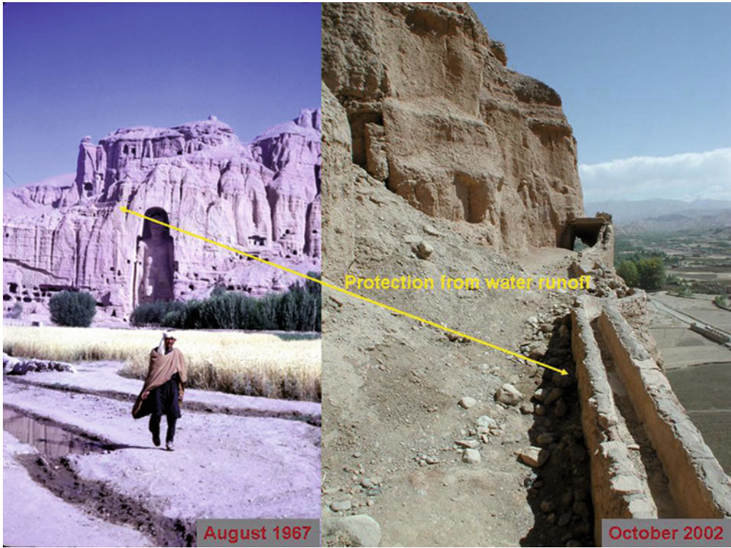
Fig. 9.7 Protection from water runoff and infiltration
