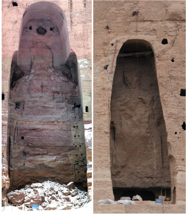
Fig. 12.1 The silhouette of statues on the back side of both niches (Western on left and Eastern on right ). At the ground of Western Buddha are the remains of the March 2001 explosion. Note the height of the western niche ( left ) is about 55 m and the eastern niche ( right ) is about 41 m (From PASCO 2003b)
