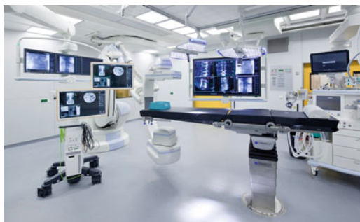
■ Fig. 17.1 Operating room set-up for computer-assisted 3D image-guided surgery
