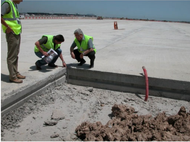
Fig. 10.28 Upper plate construction.
