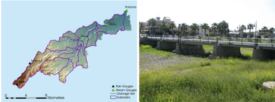
Fig. 2 Map of the catchment area indicating the subbasins, the rain and the stream gauges (left). Bridge in the downstream area of the basin where extreme inundation phenomena have taken place during 1992, 2003 and 2009 (right)
