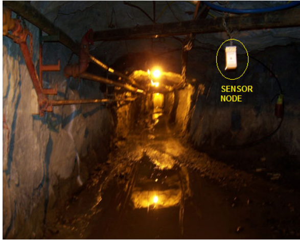
Fig. 2. Illustration of underground mine gallery and the deployment of the node (A)
