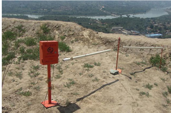
Fig. 32 An extensometer installed at a landslide in Heifangtai, Gansu province
