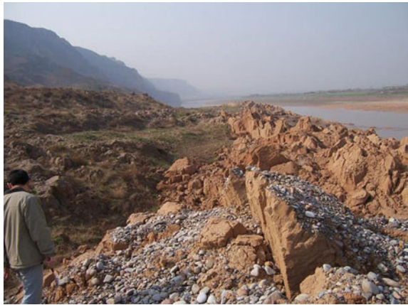
Fig. 27 The Jinghe river bed was squeezed up by the landslide
