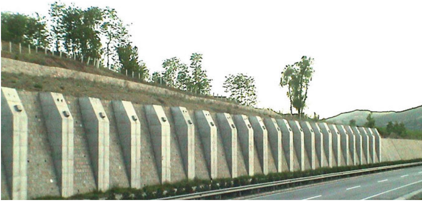
Fig. 21 The piles applied to stabilizing a landslide on the Tongchuan-Huanglin highway
