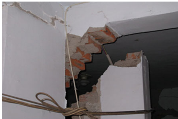
Fig. 5 The building with improper load transmission path
