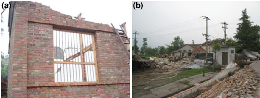
Fig. 4 The destroyed masonry timber buildings
