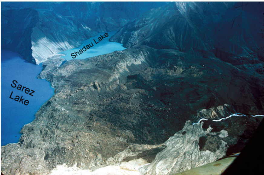
Fig. 3 The Usoi natural dam. Helicopter view from north. Giant block retaining original structure is visible on top of the dam in front of the Shadau Lake. Seeping water forms springs at the left bank of the erosion canyon. Whitish flat area above the canyon—deposits of debris flows that came in this direction before their diversion towards the Lake in 1947. Steep scarp that crosses the dam body indicate its transverse spreading likely due to impact over the steep opposite slope of the Murgab River valley
