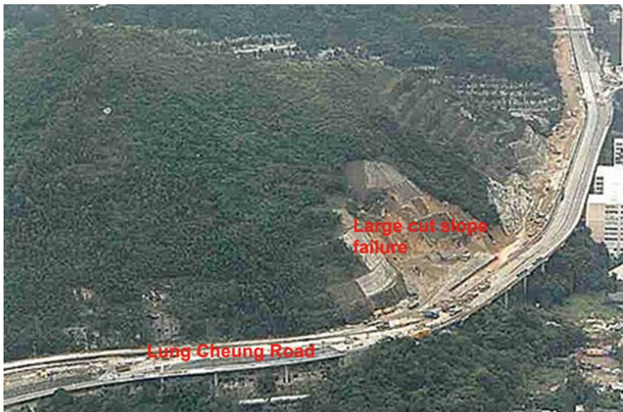
Fig. 10 Landslide in a cut slope above Lung Cheung Road in 1997 (modified after GEO)
