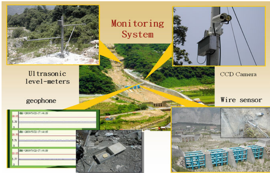
Fig. 6 Standard SWCB monitoring system. Equipments include CCD camera, geophone, wire sensor and ultrasonic level-meter, installed at Fengqiu debris-flow potential stream in the Chenyoulan stream watershed,Taiwan
