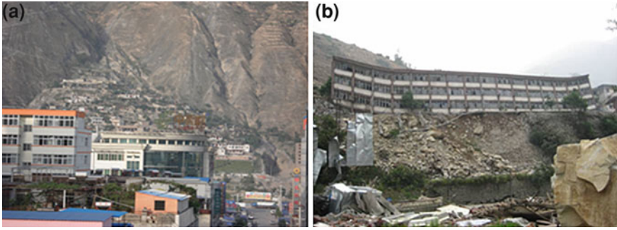
Fig. 16 The buildings built on improper location
