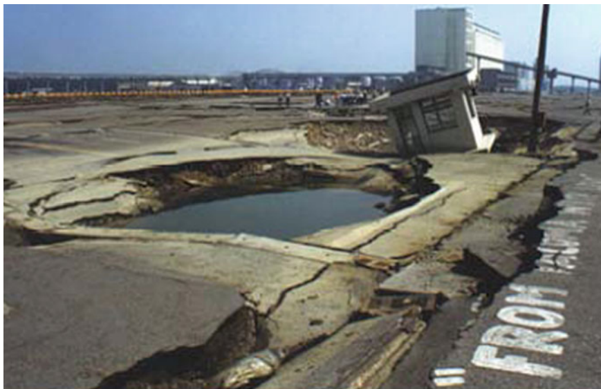
Fig. 9 Damage of Taichung port by liquefaction
