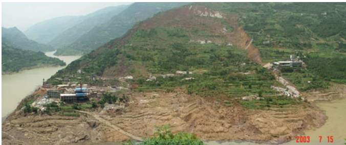
Fig. 2 Front-on view of the Qianjiangping landslide (Taken by Zhang, July 15, 2003)
