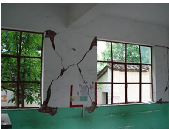
Fig. 12 The phenomenon of ‘strong beam-weak column’
