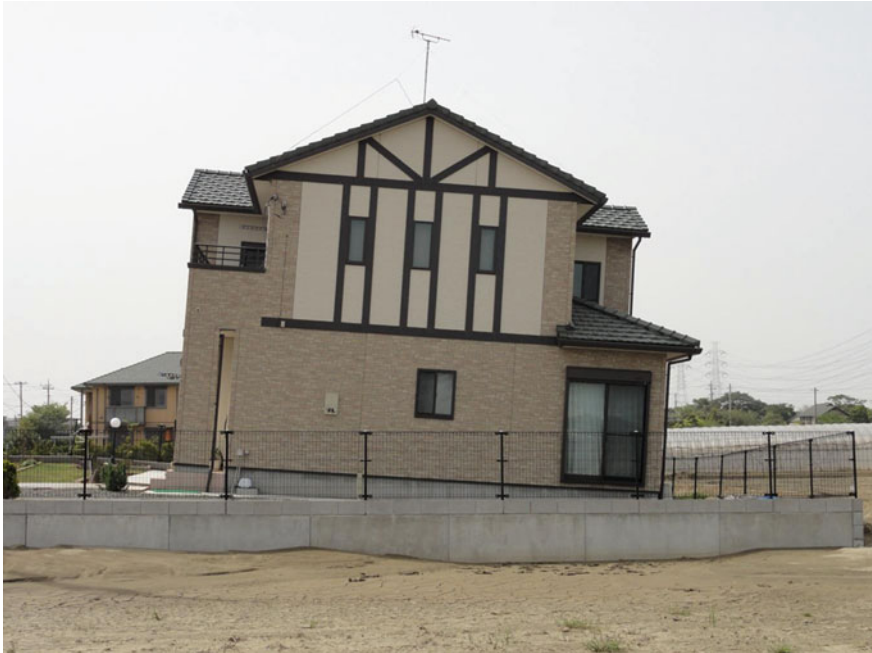
Photo 1 Damage to house by soil liquefaction
