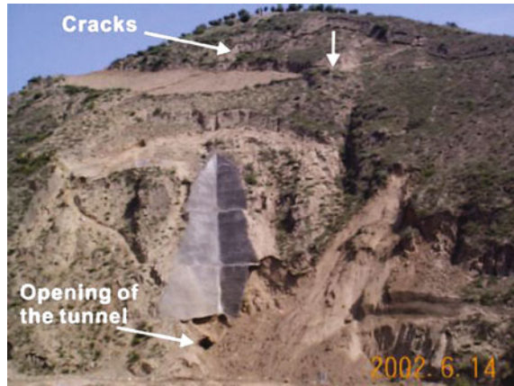
Fig. 24 Collapse and slide occurred in the opening as the tunnel being driven after a heavy rain
