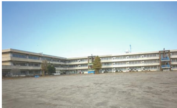
Fig. 8 School buildings are commonly taken as vertical evacuation structures but some of them have been overtopped during tsunami inundation on March 11, 2011
