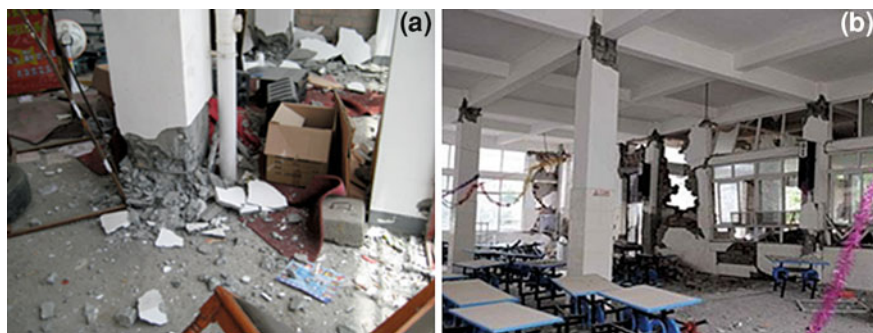
Fig. 12 The phenomenon of ‘strong beam-weak column’
