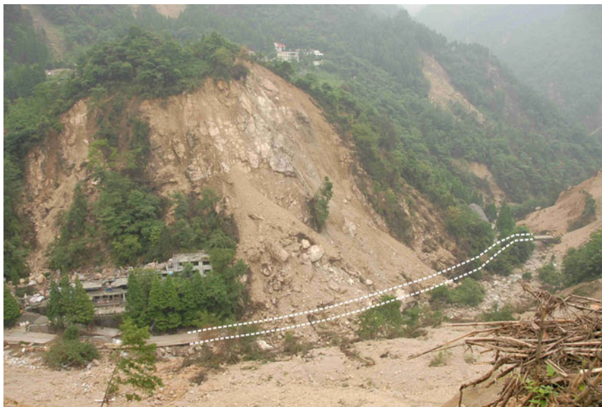
Fig. 2 This rockfall occurred in Hongyan Resort Village, located on an old landslide dam. The dashed white line shows where the road existed before the landslide
