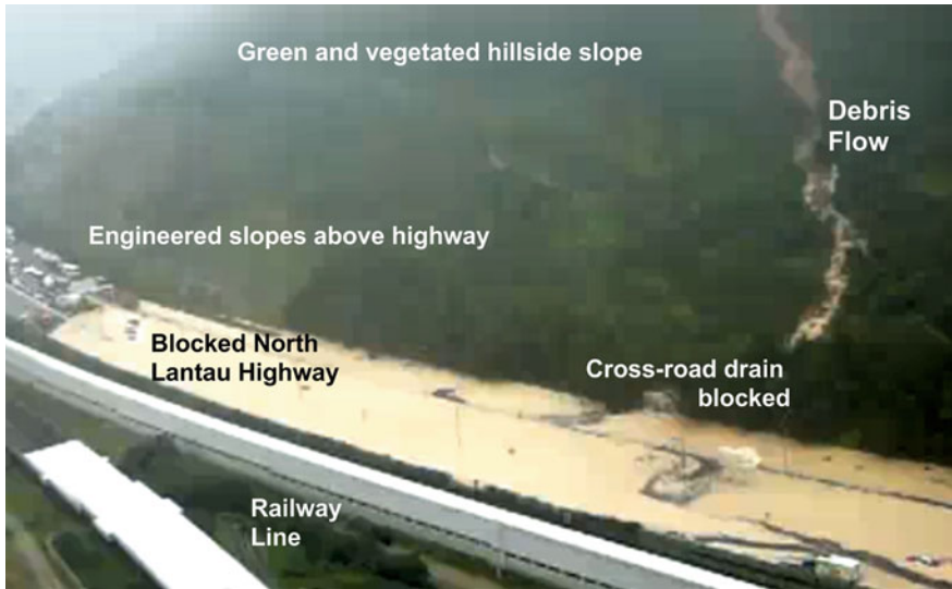
Fig. 11 Blockage of newly constructed North Lantau Express by channelized debris flow on streams from above mountain on June 7, 2008 (modified after web video)
