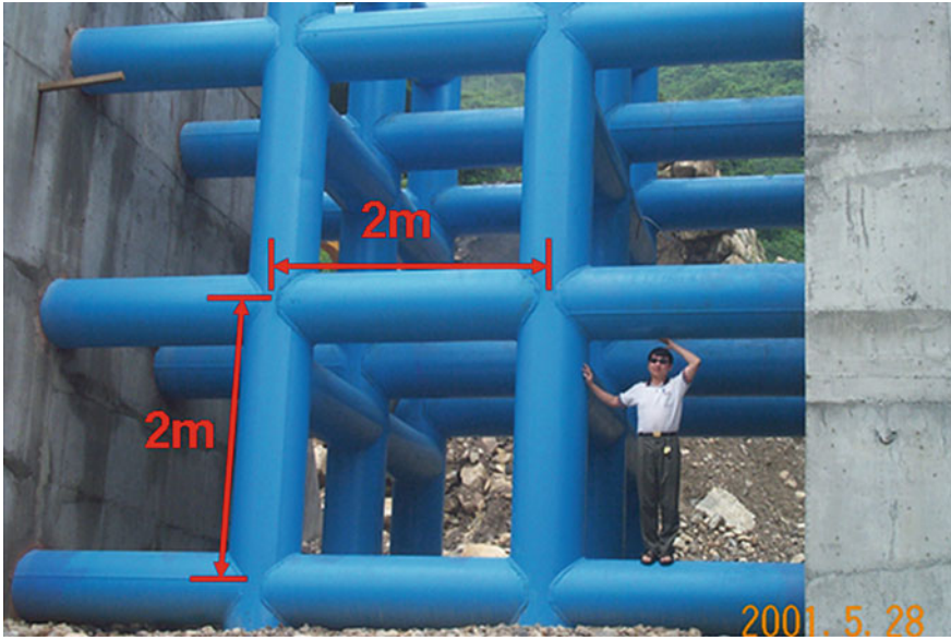
Fig. 11 Typical dimension of open-type sabo dams: steel slit dam
