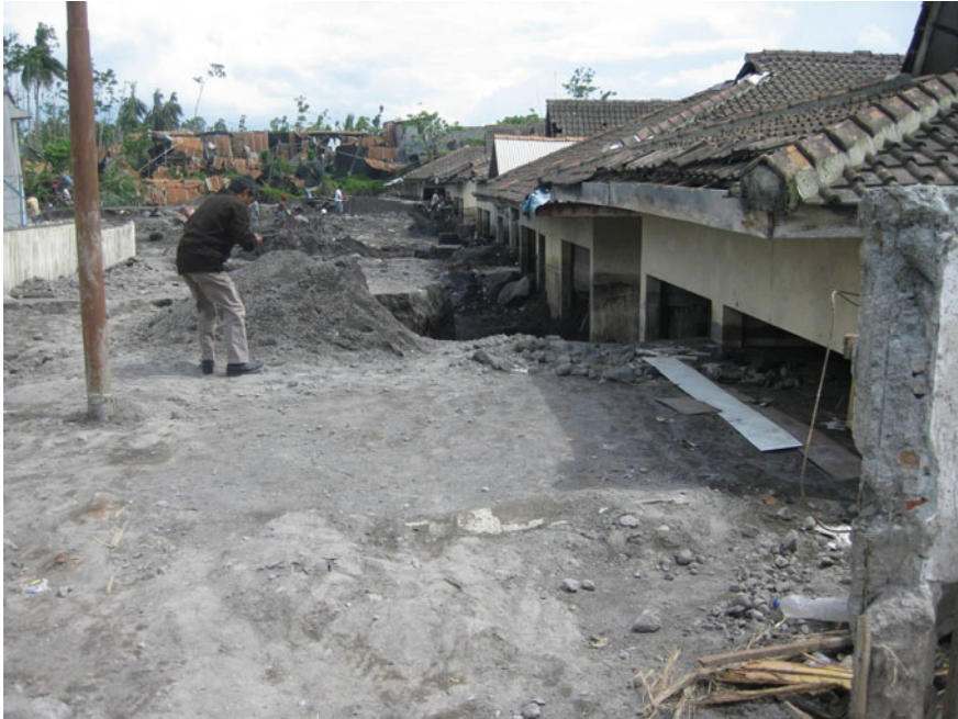
Fig. 3 Damage on houses near the volcanic river
