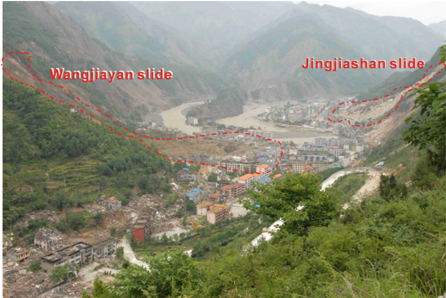
Fig. 5 The Wangjiayan earth fall/slide ( left ) and the Jingjiashan rockfall ( right ) in Beichuan county town. The Wangjiayan landslide killed 1,600 people and the Jingjiashan landslide killed 400 people. The dashed lines show the travel path and the extent of each landslide
