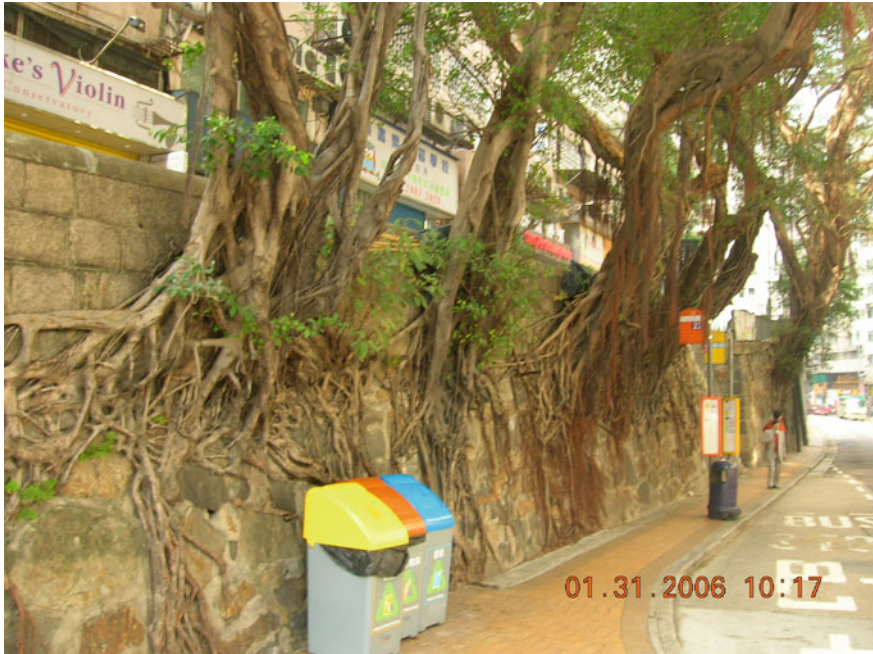
Fig. 4 Large banyan trees growing out of old masonry retaining walls on Bonham Road, Hong Kong Island
