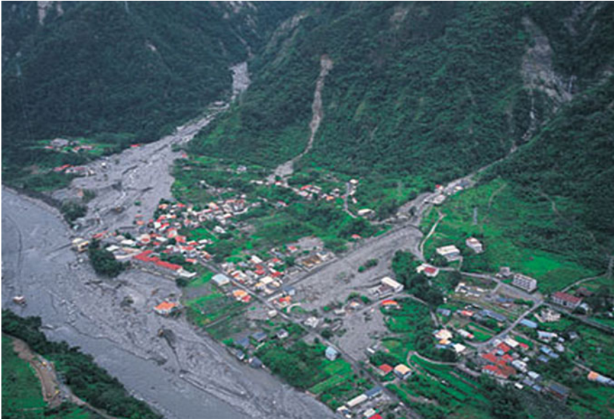
Fig. 1 Debris flow disaster at Song-Her village in central Taiwan. The village is partially buried by debris flows and an original small stream outbursts into debris flow river of more than 30 m wide. This scenario is typical in Taiwan
