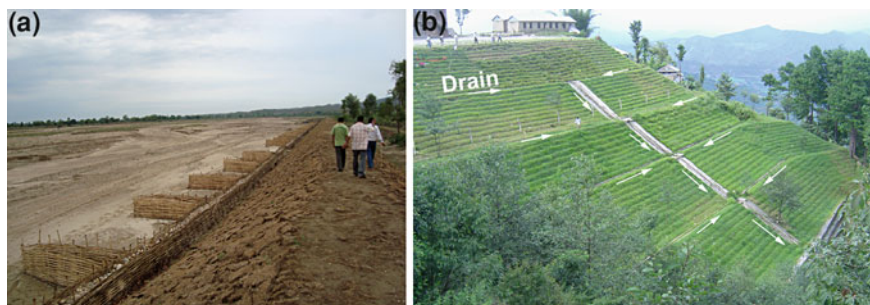
Fig. 22 a Community based river training work with bioengineering systems for flood protection in Terai and b Bioengineering work for the protection of problematic slope in a settlement area, east of Kathmandu
