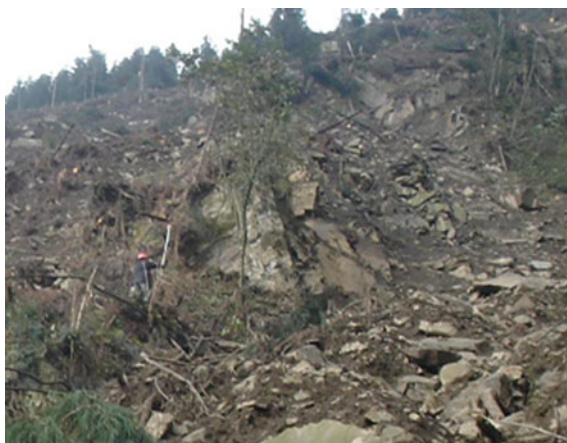
Fig. 4 Unstable rock No. 4
