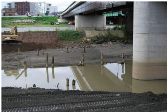
Photo 4 Former wood pile foundations near Kida Bridge
