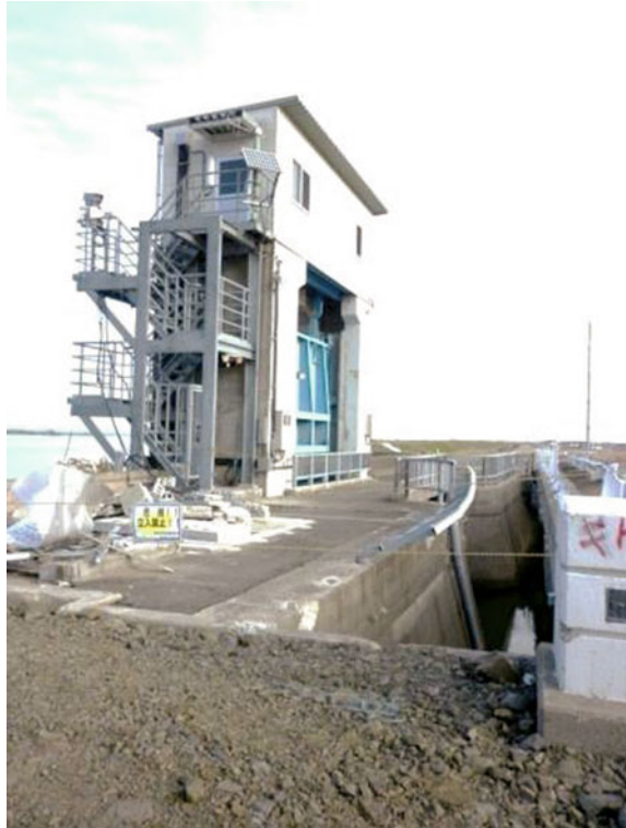
Fig. 7 Watergate that manually or automatically closed during tsunami warning
