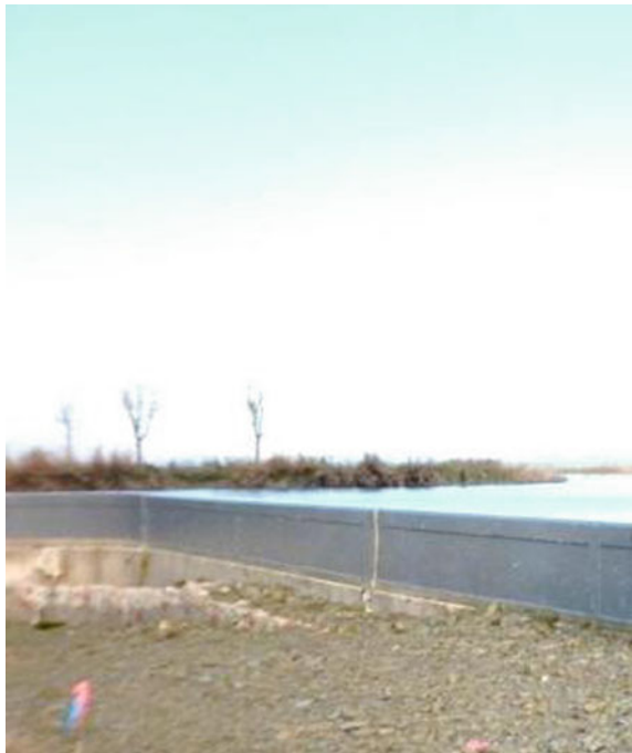
Fig. 6 Fixed tsunami seawall that have been overtopped during March 11, 2011 tsunami
