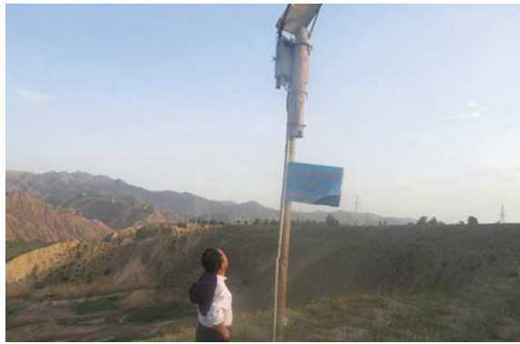
Fig. 33 A borehole inclinometer installed at a landslide in Heifangtai, Gansu province
