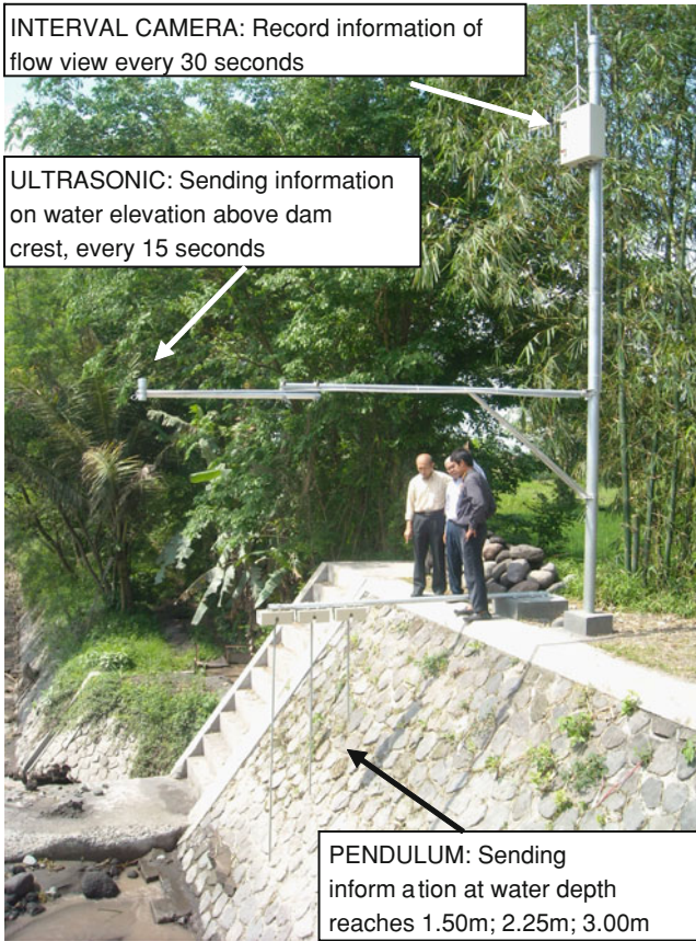
Fig. 12 Cross-sectional monitoring system at Rejodani
