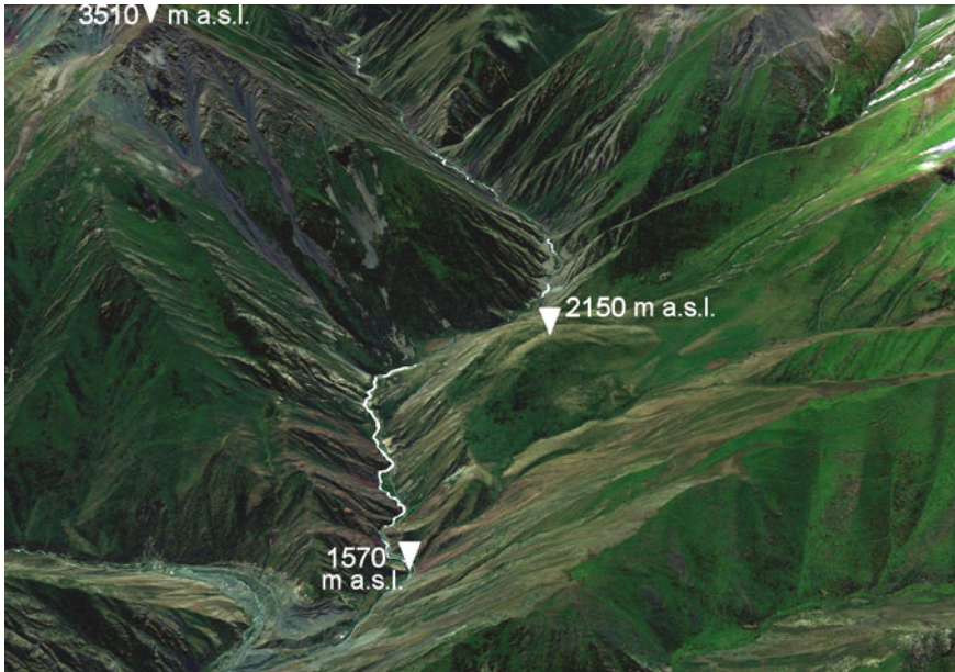
Fig. 22 Breached Aksu dam in the Aksu River valley at the northern slope of the Kyrgyz Range. Remaining part of the dam's body is the smooth hill with top mark at 2150 m a.s.l. 3D Google Earth view
