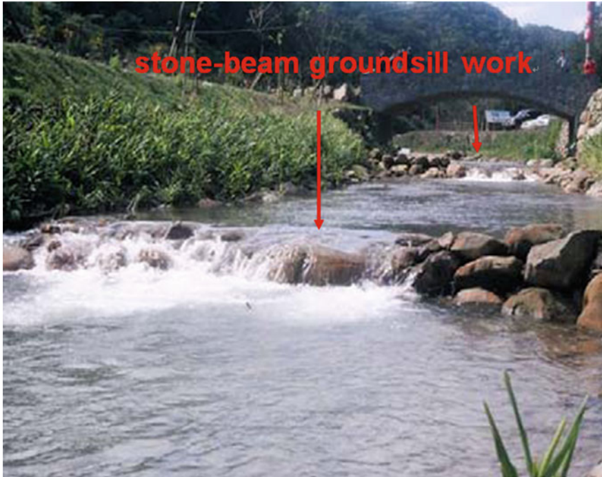
Fig. 16 Continuous stone-beam ground sill work (Hsieh 2008)
