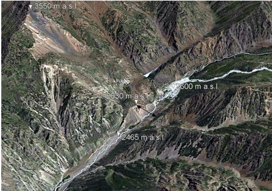
Fig. 7 The Yashinkul dam breached in 1966. Note large difference of the benchmarks elevations upstream and downstream from the dam resulting from the significant sedimentation of the 300-years old lake (compare with the Aini landslide dam on Fig. 6). Just downstream from the dam evidence of valley aggradation are still visible. 3D Google Earth view
