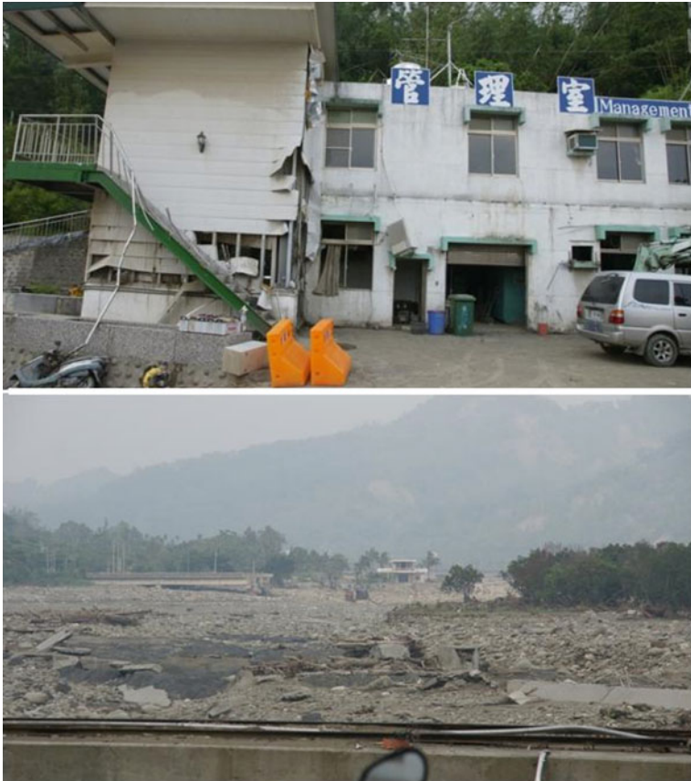
Fig. 7 Flood destroyed Chiahsien dam operation center ( top ) and nearby bridges ( bottom )
