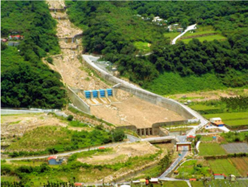
Fig. 15 Debris-flow control structures, such as Sabo dams, debris barriers, and debris basins, at Fengqiu in the Chenyoulun Stream watershed (Jan and Chen 2005)
