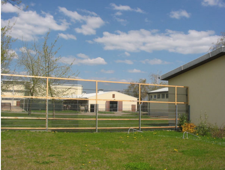
Fig. 6.3 Insecticide-treated polyester fences protect a stud bull farm in Schmergow, Brandenburg, Germany, 2009 (Rinderproduktion Berlin-Brandenburg (RBB)). The 3-m-high net consisted of black multi-filament polyester with a mesh width of 1.5 \times 1.7 mm, pre-treated with micro-encapsulated deltamethrin ( 90 \text{ mg/m}^2 ) and a UV protector
