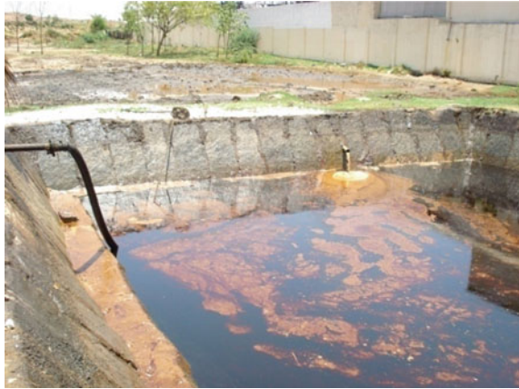
Fig. 9.3 Stagnant liquid in crude storage generates huge quantity of contaminated soil which qualifies to be solid waste
