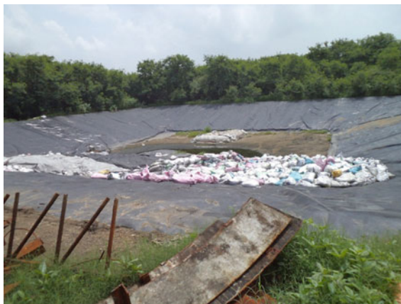
Fig. 7.17 Arrangement of non-compatible waste types in a hazardous waste disposal site
