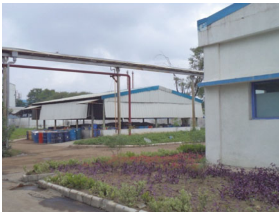
Fig. 7.7 Onsite storage of hazardous waste at an industry
