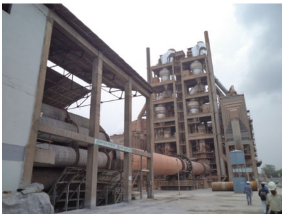
Fig. 7.16 A Cement Kiln
