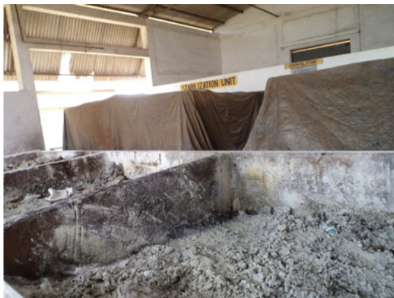
Fig. 7.12 Mixing platforms at a TSDF site
