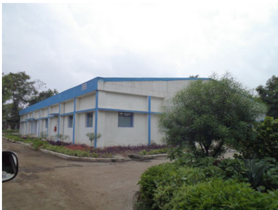
Fig. 7.8 Onsite storage of hazardous waste with a closed structure
