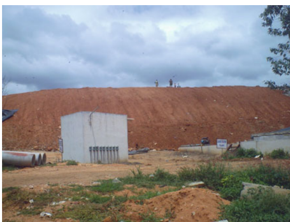
Fig. 5.14 Covering clay with topsoil in landfill cap
