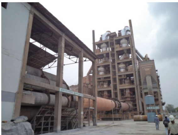
Fig. 7.16 A Cement Kiln
