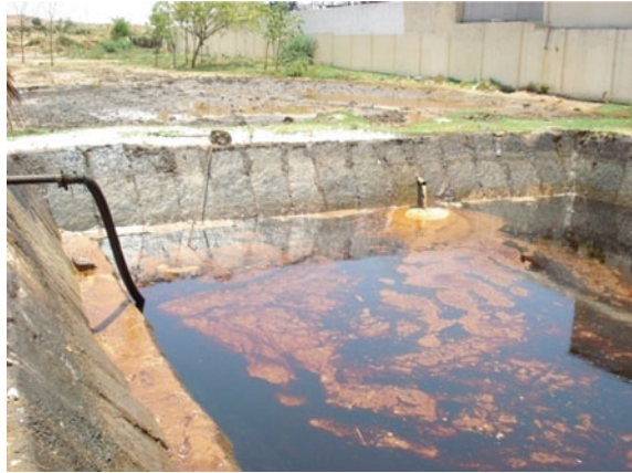
Fig. 9.3 Stagnant liquid in crude storage generates huge quantity of contaminated soil which qualifies to be solid waste
