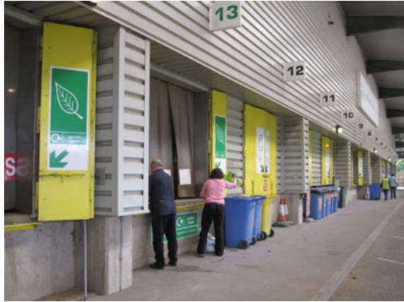
Fig. 4.1 Sophisticated waste reception at a waste processing plant
