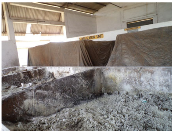
Fig. 7.12 Mixing platforms at a TSDF site
