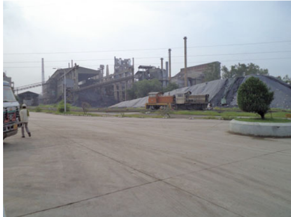
Fig. 5.15 Waste stored in a cement manufacturing facility for co-processing
