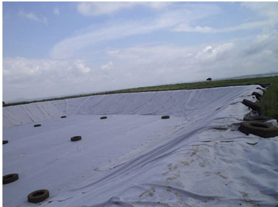
Fig. 5.9 Geotextile in Land fill area
