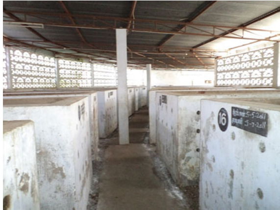
Fig. 4.34 Composting tanks
