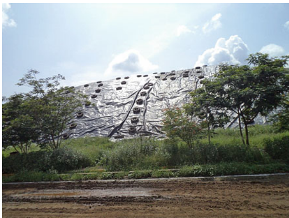
Fig. 5.12 Protection of solids filled in landfill from rain prior to capping
