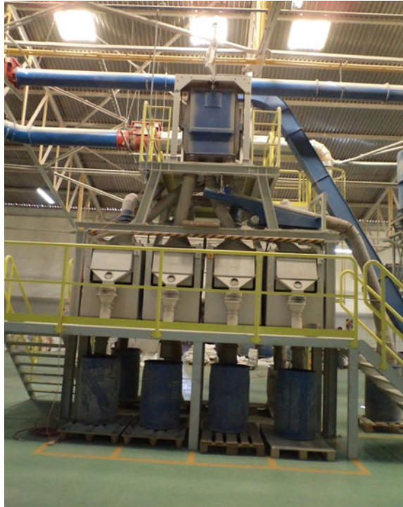
Fig. 4.17 Vibratory screen with electro static separator and collection mechanism in a WEEE processing unit
