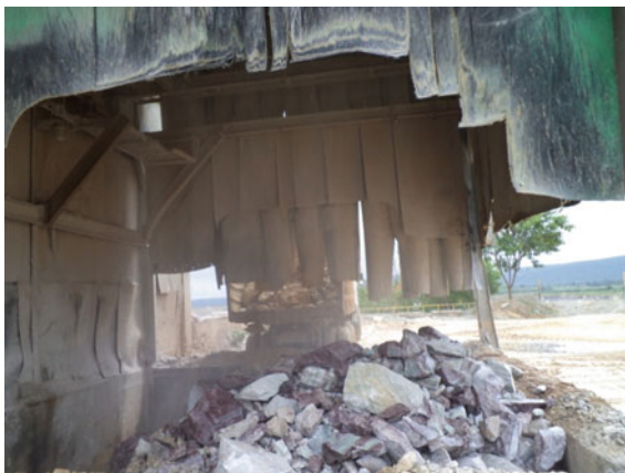
Fig. 9.7 Crusher feeder at a quarrying unit
