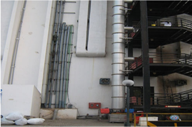
Fig. 6.6 Chute conveyor in modern hospital to transfer waste from individual wards in different floors to centralized storage area from where different category of waste will be collected and transported to common treatment facility
