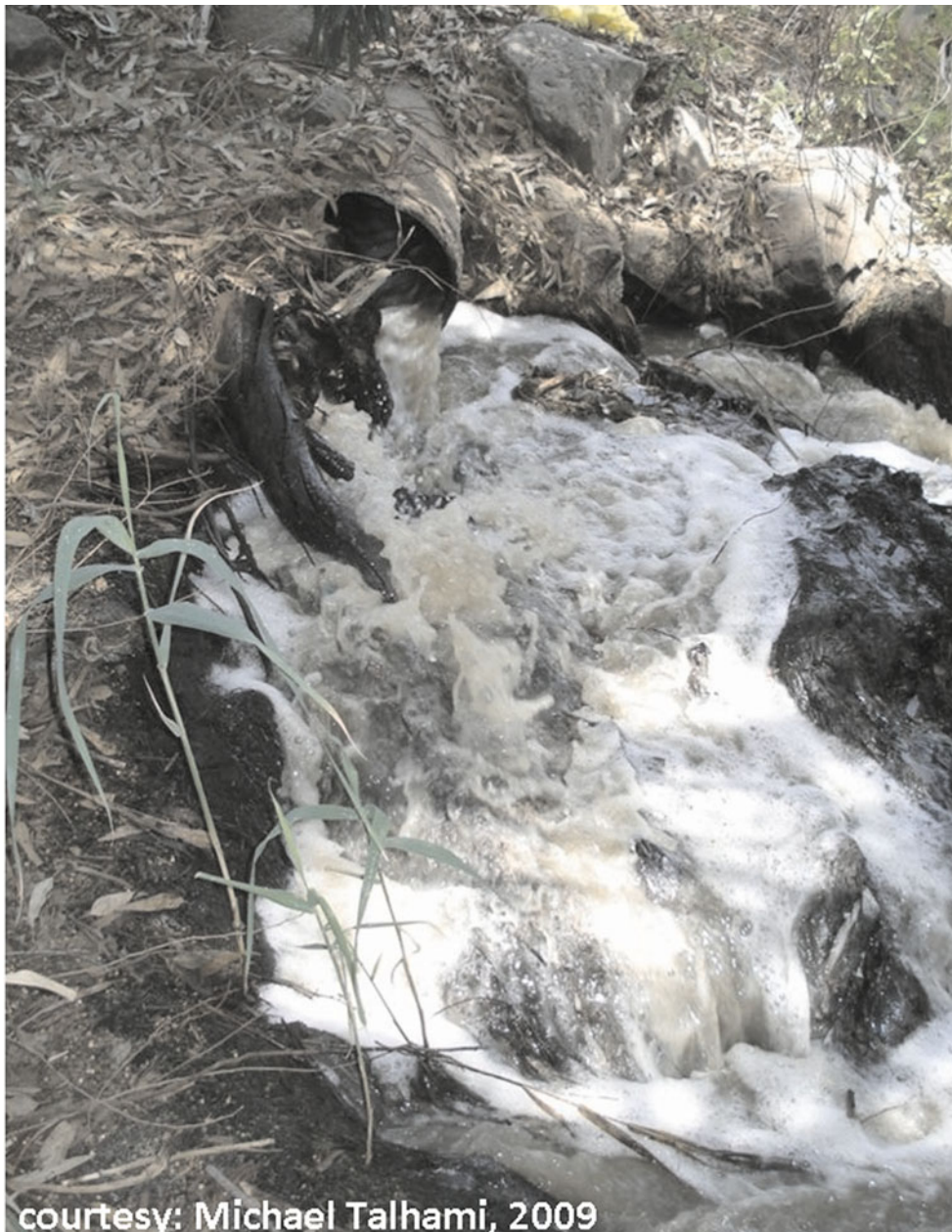
Figure 22.9: The entire Lower Jordan River at the Alumot Dam (Dagania) consisting of two pipes with raw sewage (photo) and salt bypass. Source: This figure is reproduced with permission by Michael Talhami.
