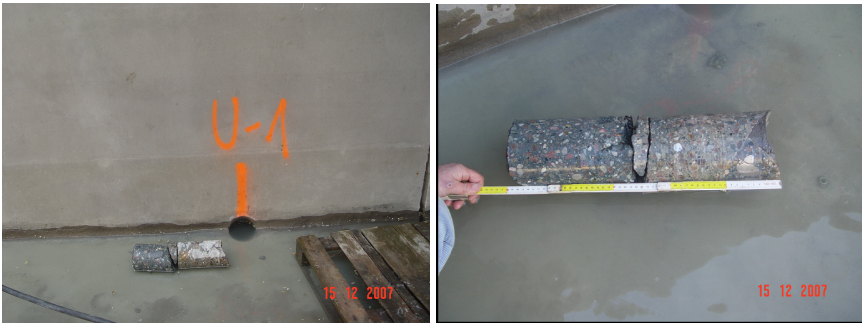
Fig. 7.91 Concrete samples taken from wall corner (Bobiński and Tejchman 2009)
