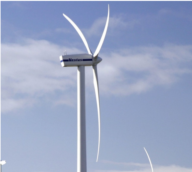
Fig. 6.31. Vestas V80 at full power with greatly deflected rotor blades
