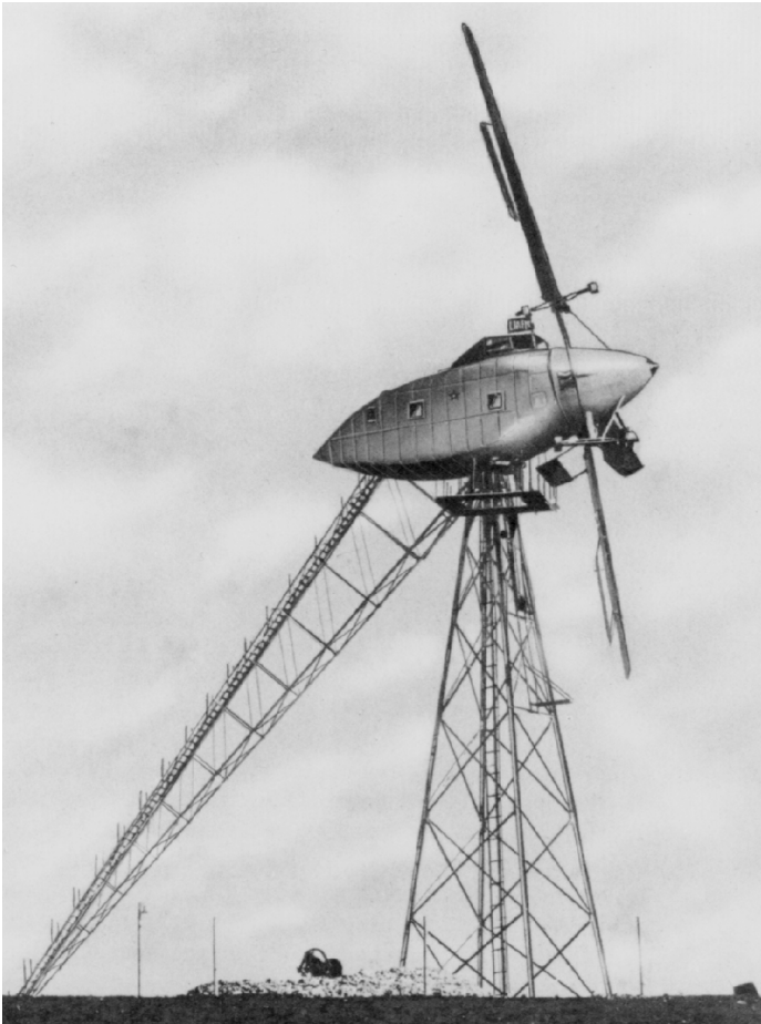
Fig. 2.8. Russian wind turbine WIME D-30 in Balaklava on the Crimea (rotor diameter 30 m, rated power approx. 100 kW), 1931
