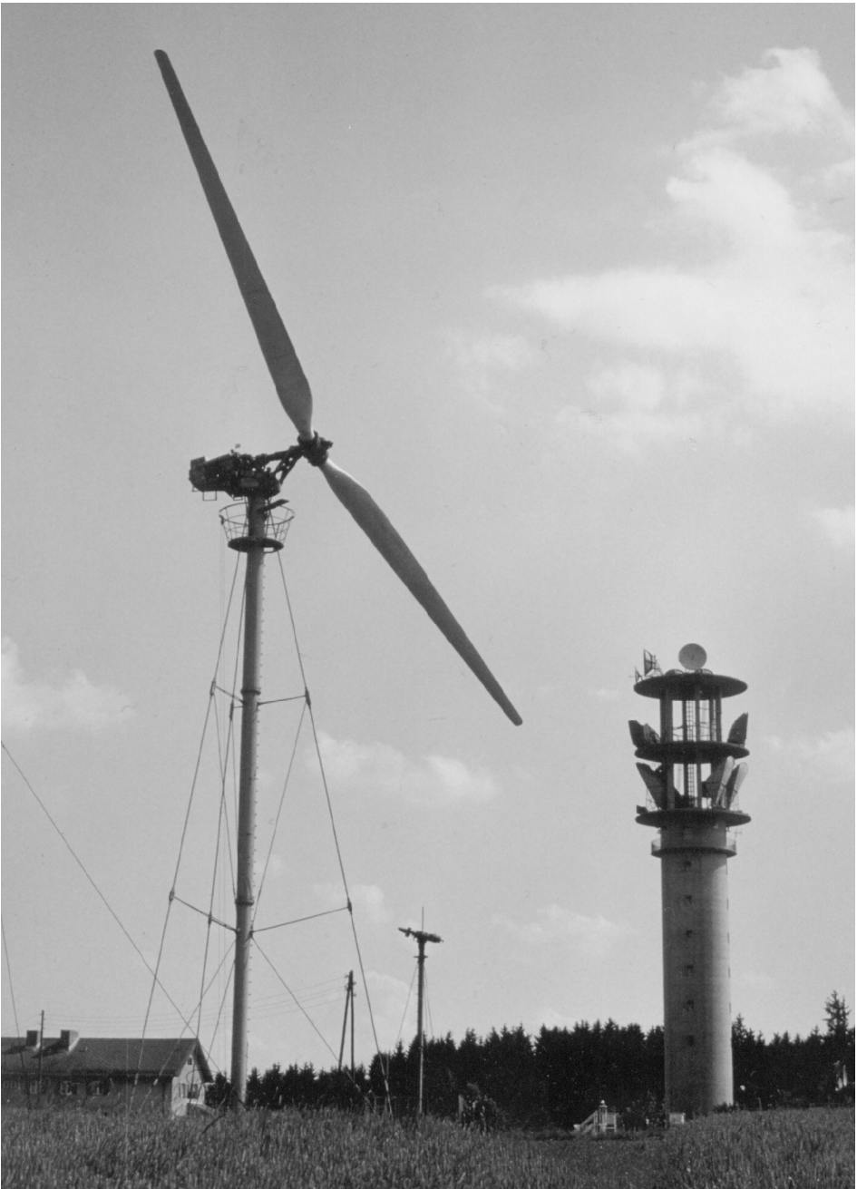
Fig. 2.16. W-34 wind turbine by U. Hütter in Stötten in the Swabian Alb, Germany (rotor diameter 34 m, rated power 100 kW), 1958-1968
