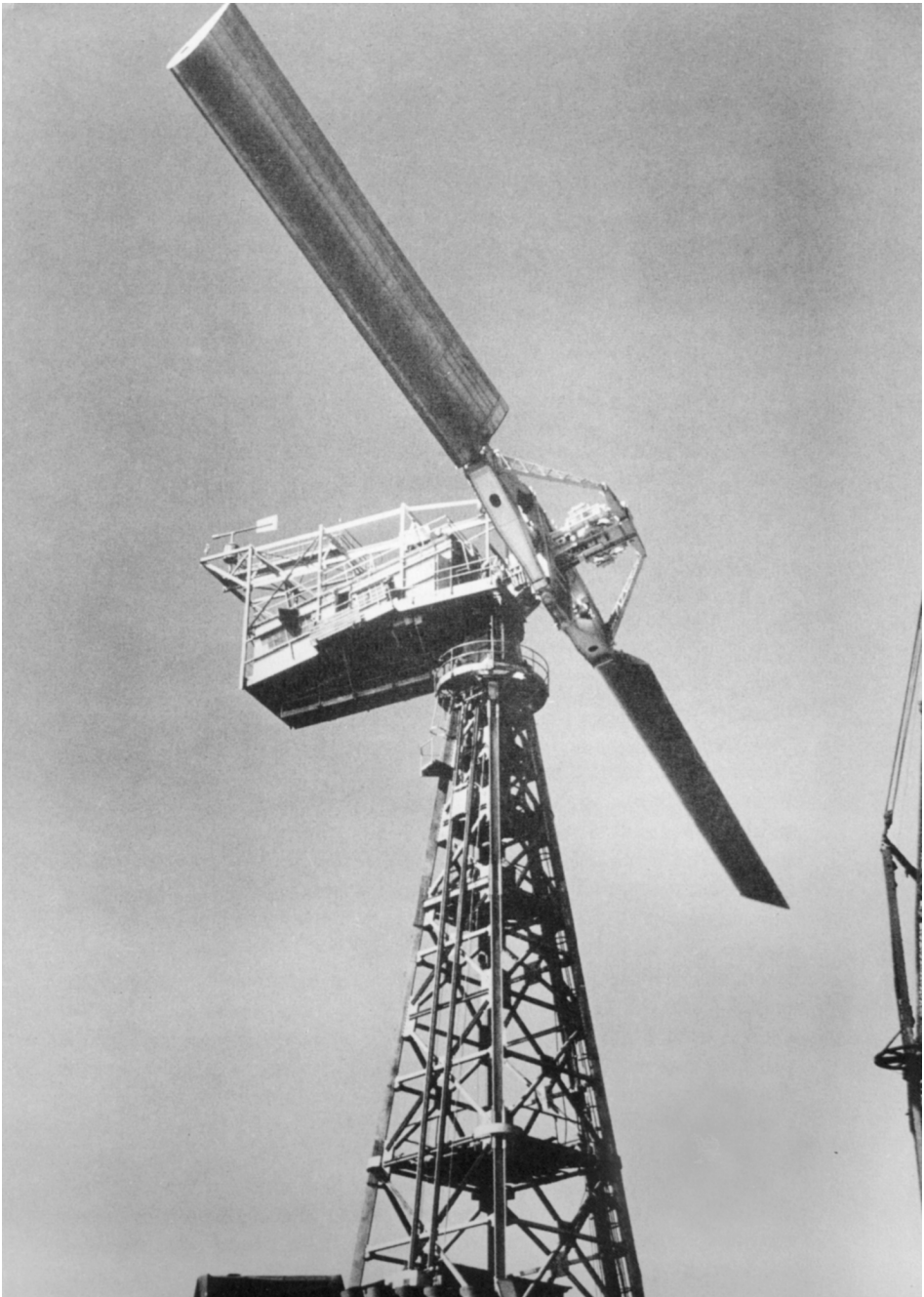
Fig. 2.10. Smith-Putnam wind turbine, in Vermont, USA. (rotor diameter 53.3 m, rated power 1250 kW), 1941 [15]
