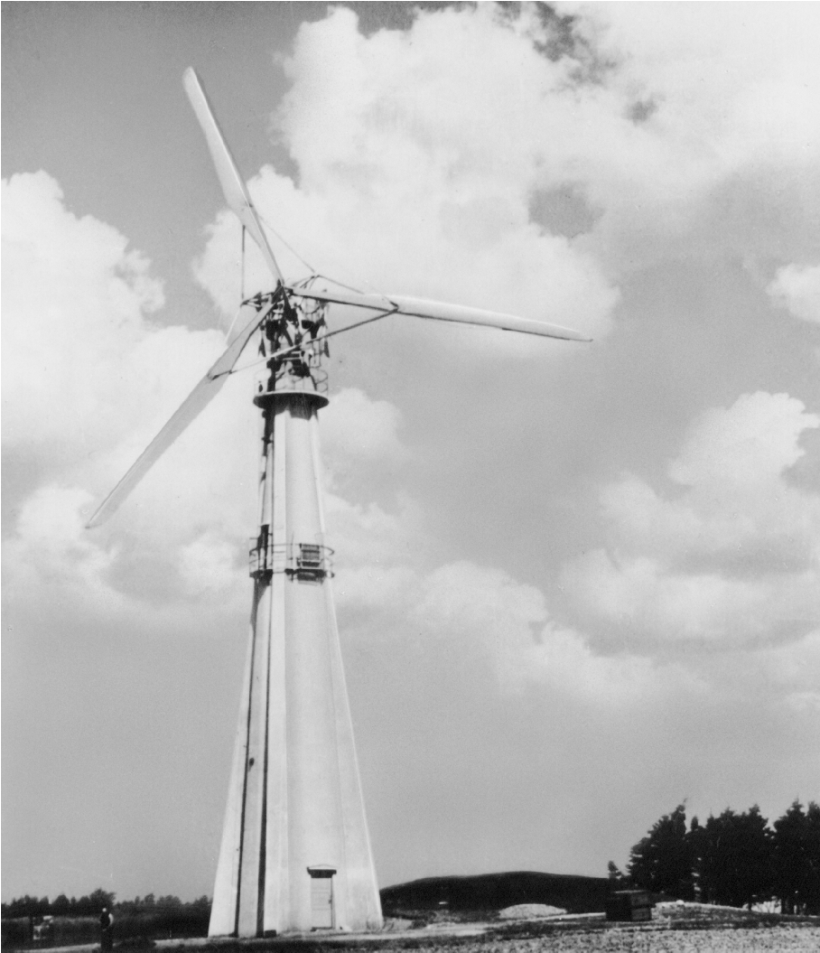
Fig. 2.5. Smidth "Aeromotor" with three-bladed rotor (rotor diameter 24 m, rated power approx. 70 kW), 1942 [5]
