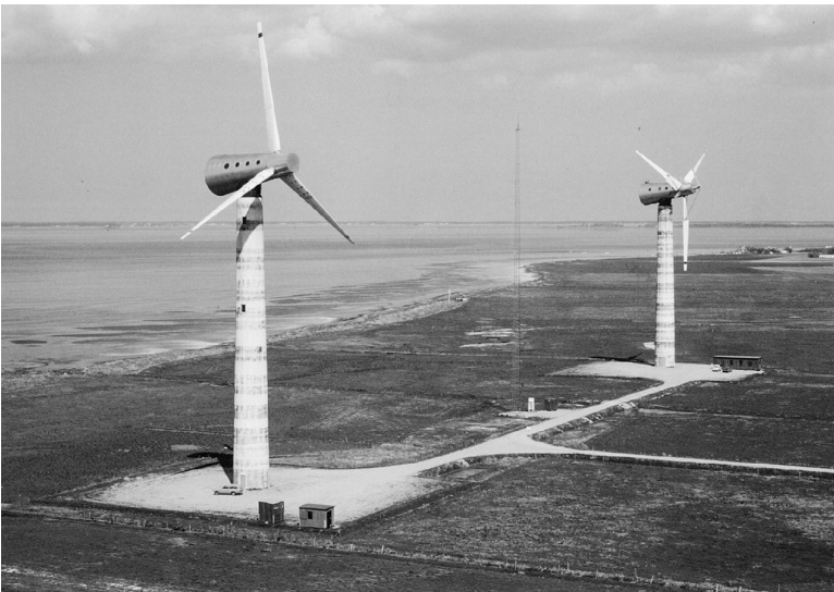
Fig. 2.24. Nibe A and Nibe B, (rotor diameter 40 m, 630 kW), ELSAM (Denmark), 1979
