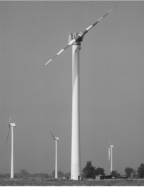
Fig. 2.29. Aeolus II in Wilhelmshaven, Germany, (rotor diameter 80 m, 3000 kW), three Monopteros in the background, 1990
