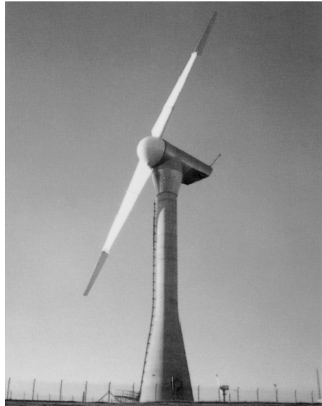
Fig. 2.35. LS-1 (rotor diameter 60 m, 3000 kW), WEG (United Kingdom), 1988
