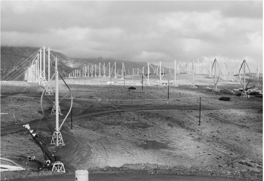
Fig. 2.46. Flowind wind farm with vertical axis Darrieus turbines on the Tehachapi Mountains, 1986
