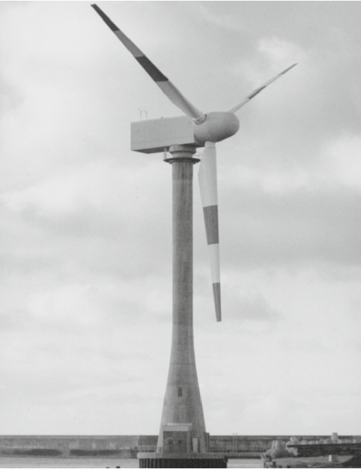
Fig. 2.30. WKA-60 on Heligoland, Germany, (rotor diameter 60 m, 1200 kW), 1993
