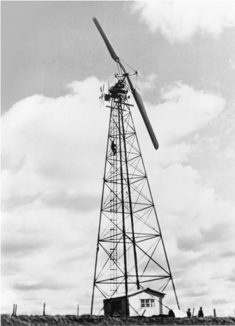
Fig. 2.3. Smidth "Aeromotor" (rotor diameter 17 m, rated power approx. 50 kW), 1941 [5]
