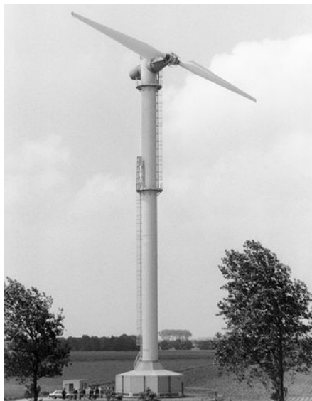
Fig. 2.37. NEWECS-45, (rotor diameter 45 m, 1000 kW), STORK (Holland), 1985
