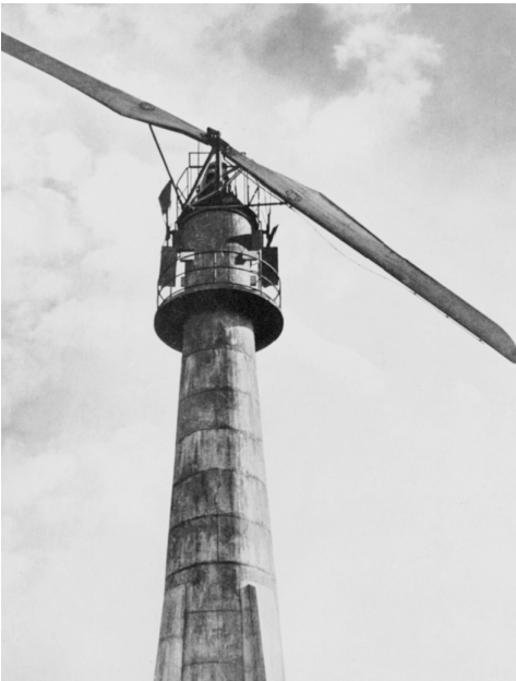
Fig. 2.4. Smidth "Aeromotor" with concrete tower (rotor diameter 17 m, rated power approx. 50 kW), 1942 [5]
