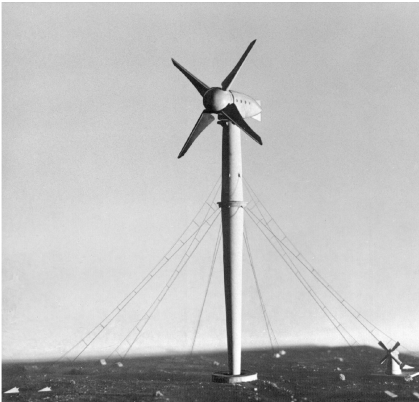
Fig. 2.7. Project MAN-Kleinhenz (rotor diameter 130 m, rated power 10 000 kW), 1942
