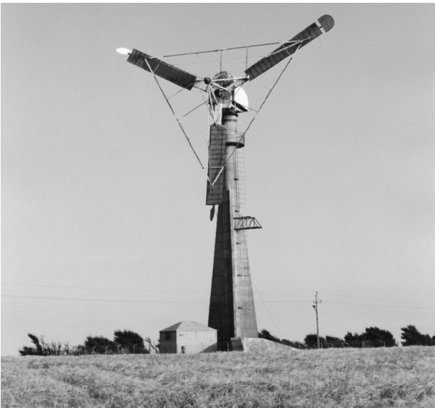
Fig. 2.15. Danish Gedser wind turbine (rotor diameter 24 m, rated power 200 kW), 1957
