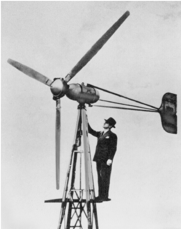
Fig. 2.9. Jacobs "wind charger" (rotor diameter about 4 m, rated power 1.8 to 3 kW), 1932
