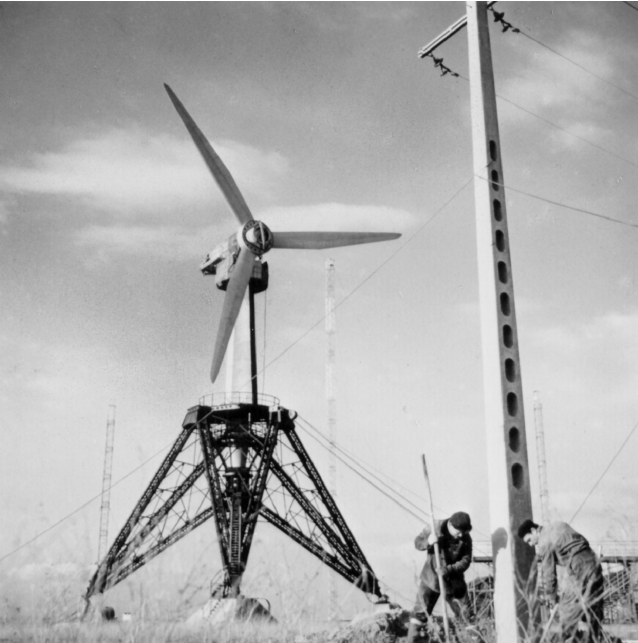
Fig. 2.13. Wind turbine by Best-Romani, France (rotor diameter 30 m, rated power 800 kW), 1958 [16]
