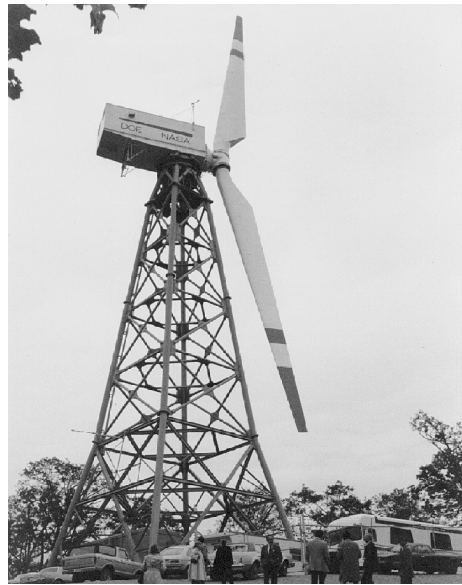
Fig. 2.19. MOD-1, (rotor diameter 60 m, 2000 kW), in Blowing Rock, North Carolina, GENERAL ELECTRIC (USA), 1979
