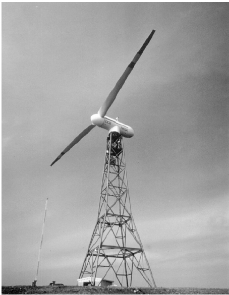
Fig. 2.18. MOD-0, (rotor diameter 38 m, 200 kW), in Clayton, New Mexico, NASA (USA), 1975
