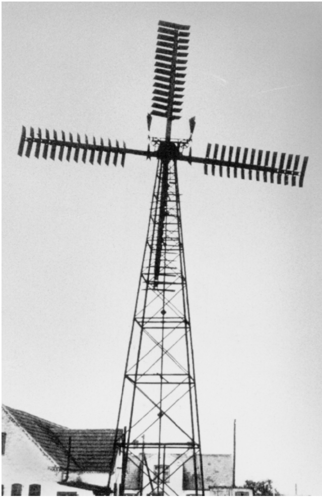
Fig. 2.2. La-Cour-Lykkegard wind turbine in Denmark. (rotor diameter 18 m, approx. 30 kW power output at 12 m/s wind speed) [4]
