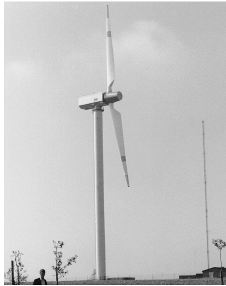
Fig. 2.32. WTS-3 (rotor diameter 78 m, 3000 kW), Swedyard (Sweden), 1982
