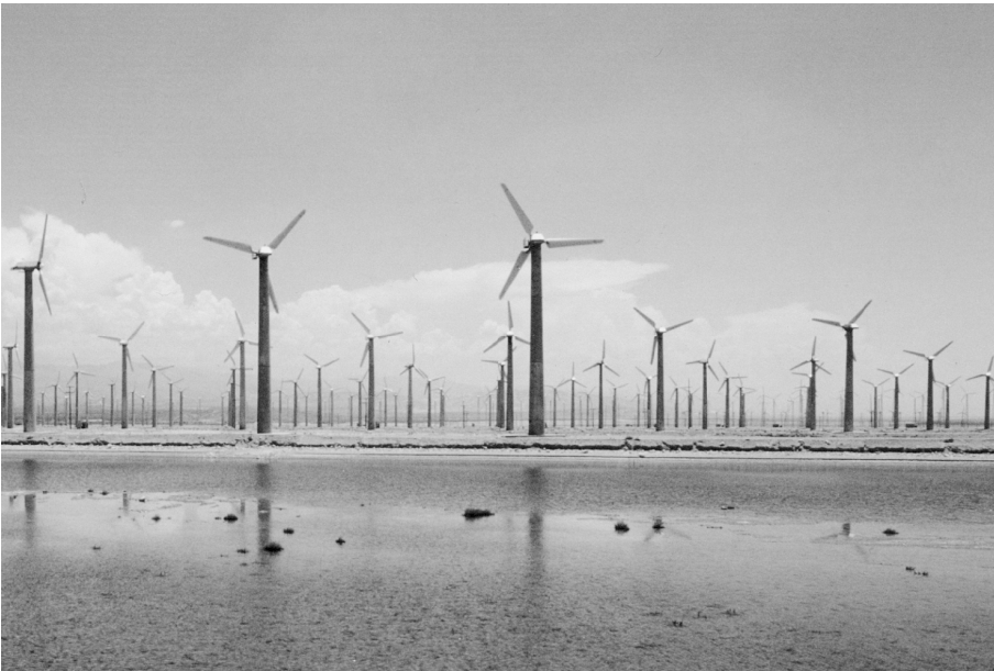
Fig. 2.44. Wind farm with Danish Micon turbines at the San Geronio Pass, 1986
