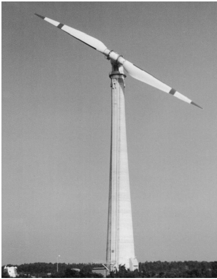
Fig. 2.31. WTS-75 (Aeolus I), (rotor diameter 75 m, 2000 kW), Kvaerner (Sweden), 1983
