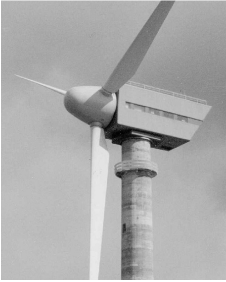
Fig. 2.38. Tjaereborg experimental turbine (rotor diameter 61 m, 2000 kW), ELSAM (Denmark), 1989
