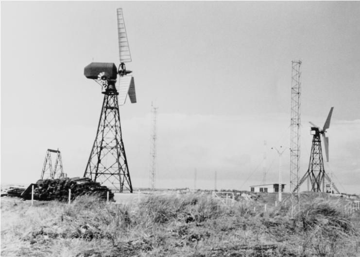
Fig. 2.14. Neypric-Vadot wind turbines in Saint-Remy: Small wind turbine (rotor diameter 21 m, rated power 800 kW); large wind turbine (rotor diameter 35 m, rated power 1000 kW), 1962-1964 [16]
