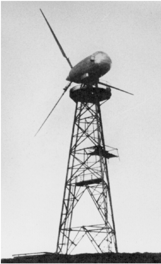
Fig. 2.11. Wind turbine of the John Brown Company on the Orkneys. (rotor diameter 15 m, rated power 100 kW), 1950 [16]
