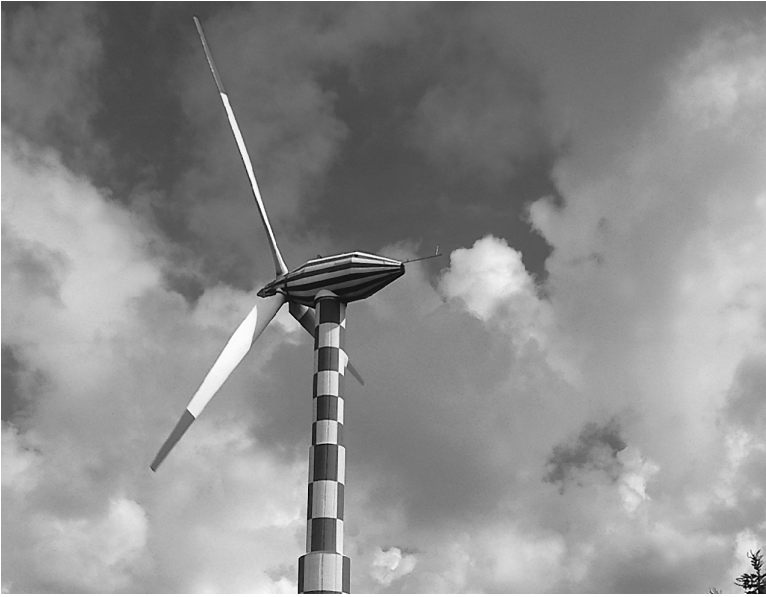
Fig. 2.23. Tvind turbine near Ulfborg, (rotor diameter 52 m, 2000 kW), (Denmark), 1978 (photo Oelker)
