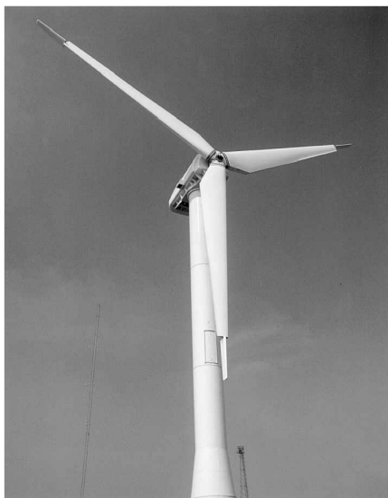
Fig. 2.36. HWP-55, (rotor diameter 55 m, 1000 kW), HOWDEN (United Kingdom), 1989
