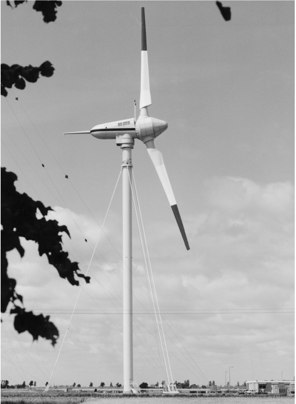
Fig. 2.25. Growian on the Kaiser-Wilhelm-Koog, (rotor diameter 100 m, 3000 kW), MAN (Germany), 1982
