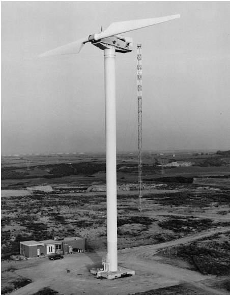
Fig. 2.34. Gamma 60 (rotor diameter 60 m, 1500 kW), AERITALIA (Italy), 1987
