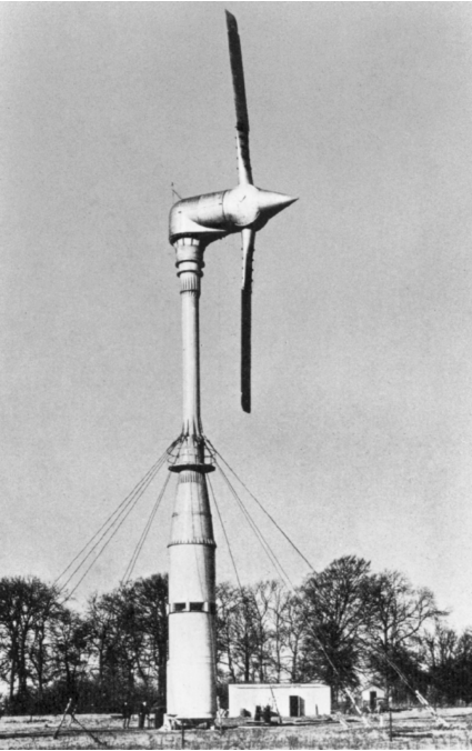
Fig. 2.12. Andreau-Enfield wind turbine in St. Albans (Hertfordshire) (rotor diameter 24 m, rated power 100 kW), 1956
