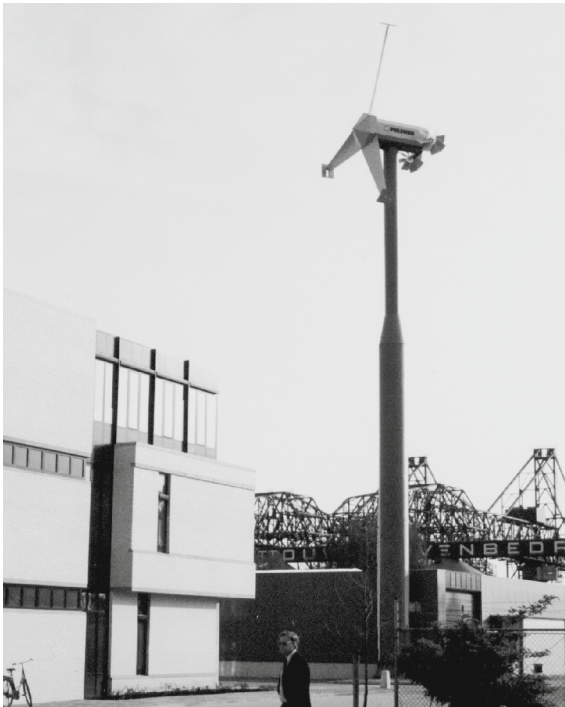
Fig. 15.16. Small wind turbine at the premises of a Dutch company
