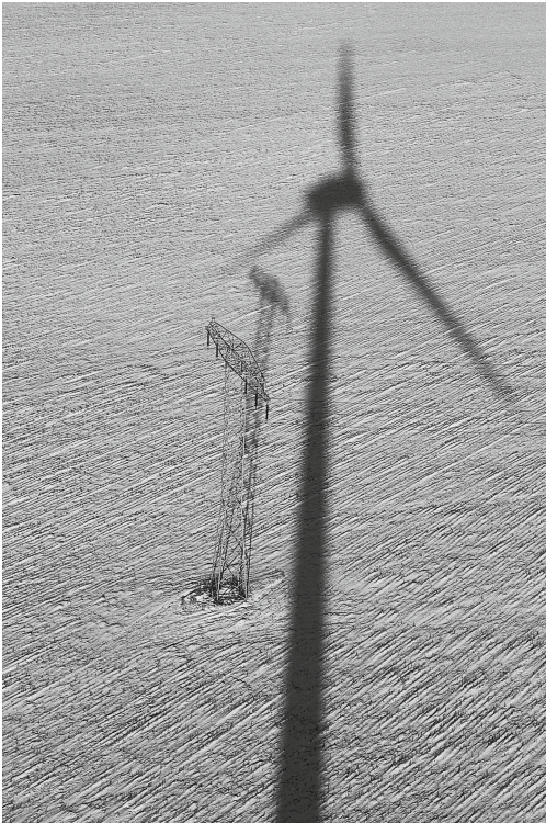
Fig. 15.11. Shadow cast by a wind turbine nearby (photo Oelker)
