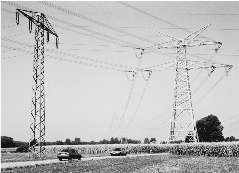
Fig. 15.19. Power transmission lines near a large town
